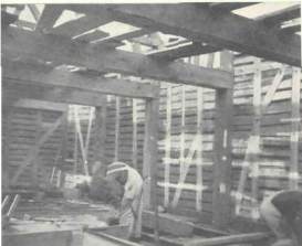
Wall Construction and Tie Beams
