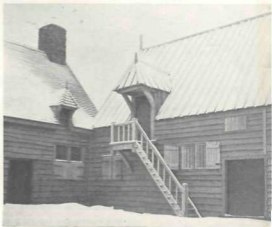
Storehouse, Looking North-East in Courtyard
