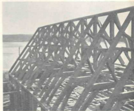
Coupled Truss Roof Construction
