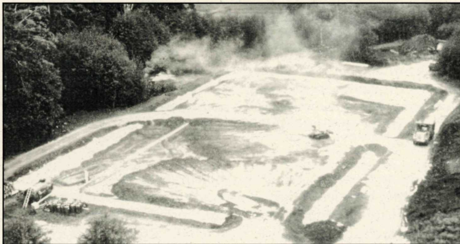
Constructing the 40m x 80m x 3m cell to hold impacted soils from various sites
