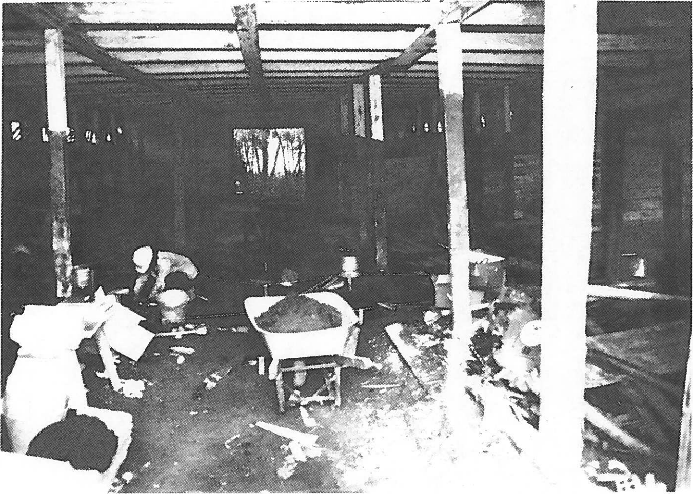
Figure 4.26. General view of excavations inside extant structure. (Photo by B. Ross.)
