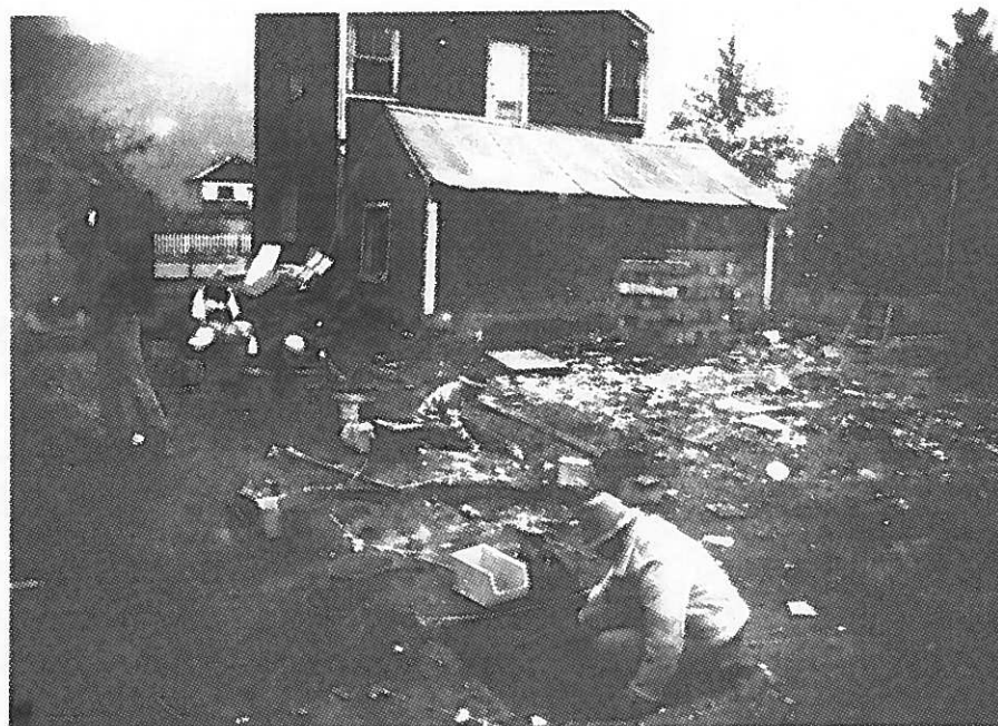
Figure 1.9. Excavations south of Annexes A and B. Note that Annex B has been moved from its original location. (Photo by B. Ross)
