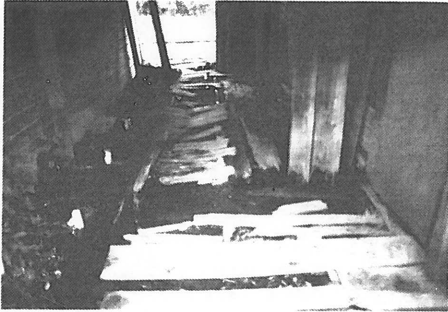
Figure 1.10. Boardwalk remains between annexes, looking north. (Photo by B. Ross)
