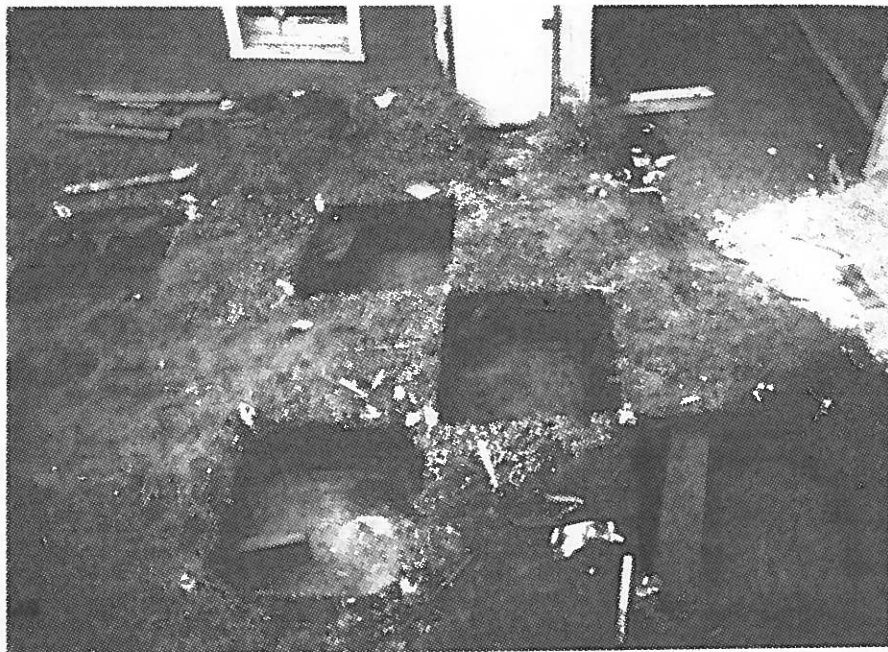
Figure 1.8. Excavations north of Annex A. (Photo by B. Ross)
