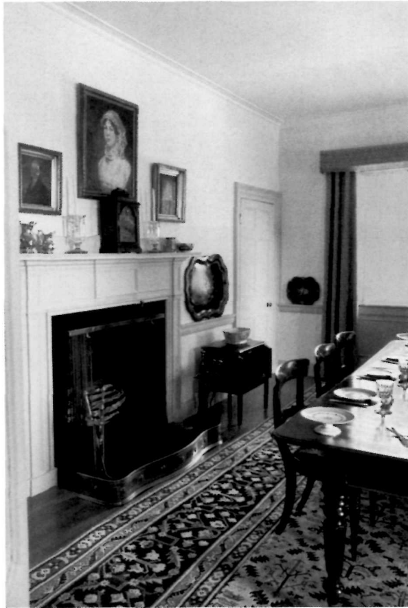
Another view of the dining room. Note the cyma reversa moulding (S-shaped with the upper part convex and the lower part concave), used here to support large plates. (Heritage Recording Services, Environment Canada — Parks, 1980)
