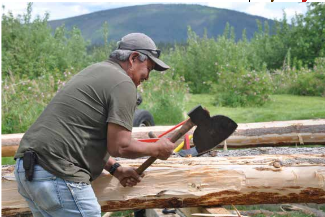
Figure 4.9: Kevin Blanchard, member of the Tr'ondëk Hwëch'in heritage crew, shaping logs at Forty Mile, 2017.
