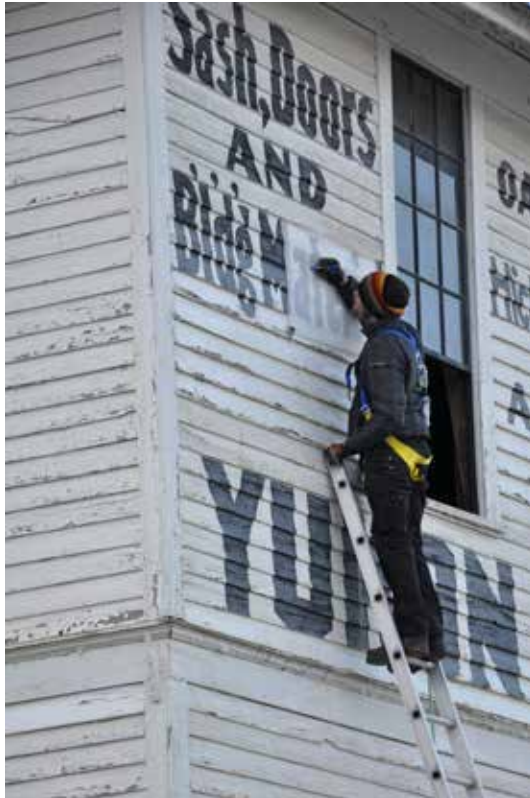
Figure 3.20: Conserving signage on Yukon Saw Mill Co. building.
