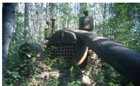
Figure 2.15: Klondike Sawmill boiler and pipe.
