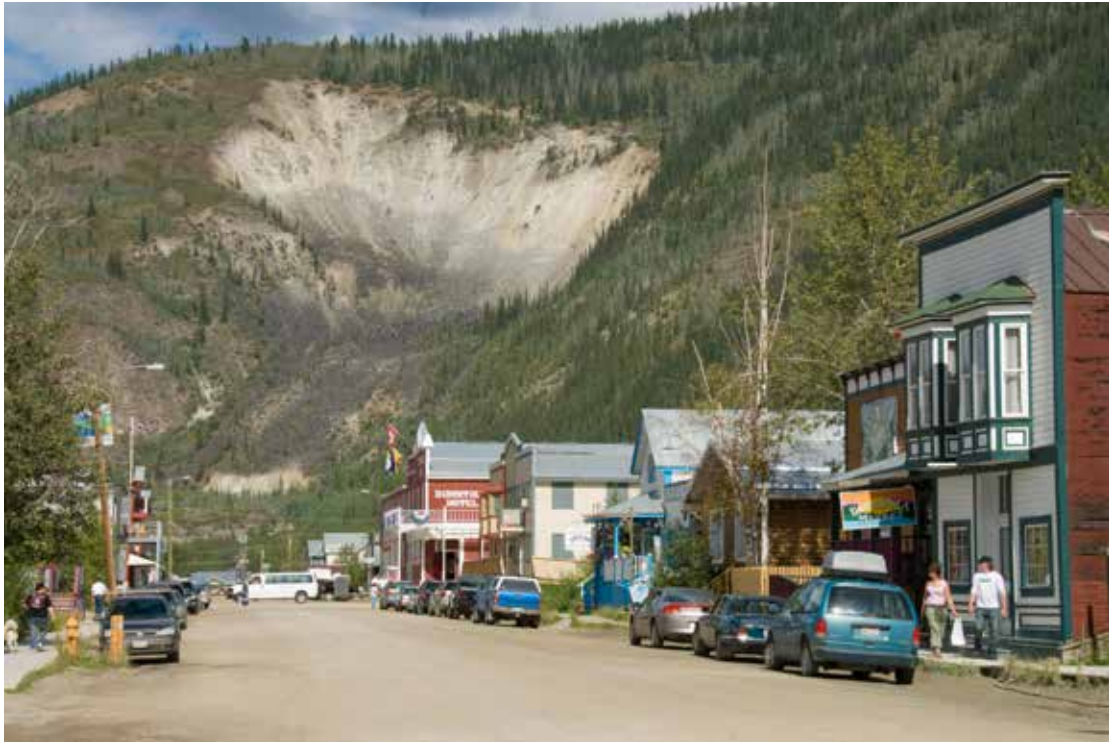
Figure 2.18: Dawson City streetscape with Moosehide Slide in background.
