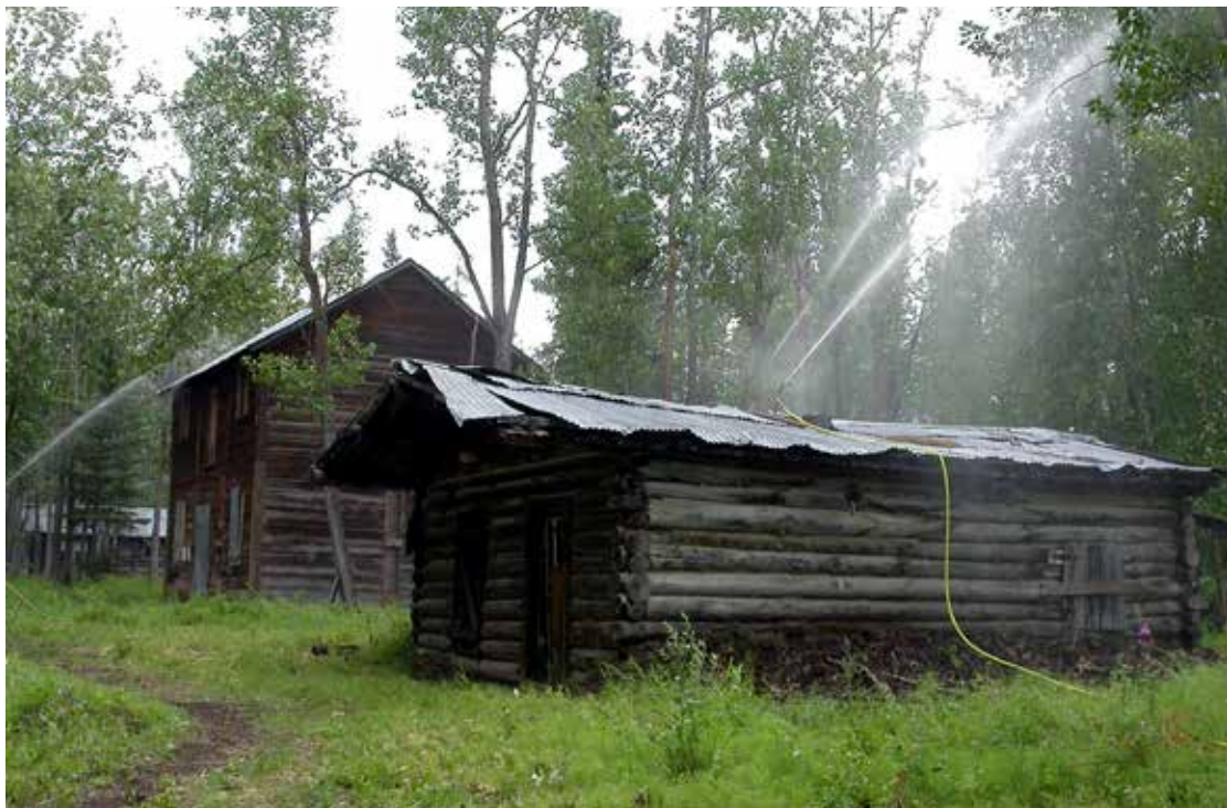
Figure 4.18: Sprinkler system at Forty Mile protecting historic buildings under threat from area wildfire, 2009.
