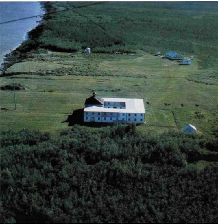
The York Factory depot is the oldest standing wooden building in Canada erected on permafrost. When this photograph was taken, it was being repainted. The small building (upper left) is the archaeologist's home; the large building (upper right) was the park superintendent's house, since destroyed by fire. Photographs are by the author.
