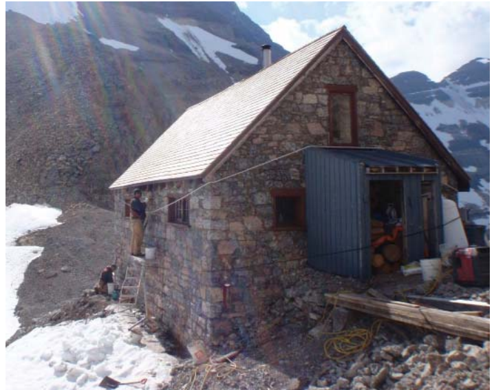
Re-pointing work underway at Abbot Pass Refuge Cabin (© Parks Canada / R. Pennell)
