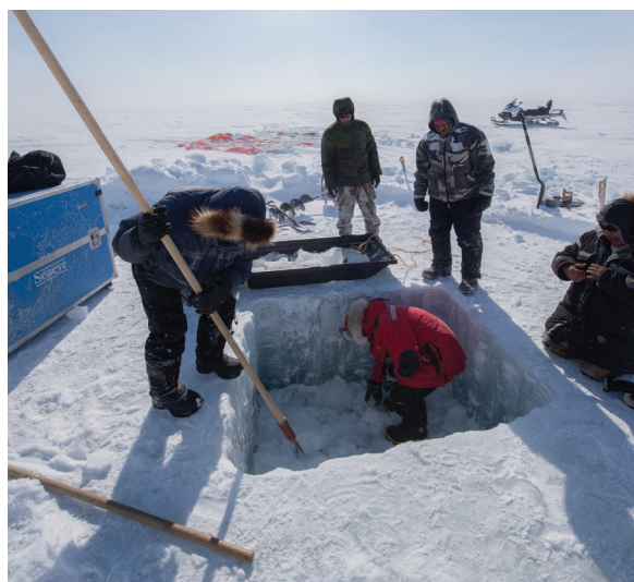
Figure 3.2.2: Excavation of the ROV access hole through thick sea ice (Photo: T. Boyer, Parks Canada; 90M00606EF).
