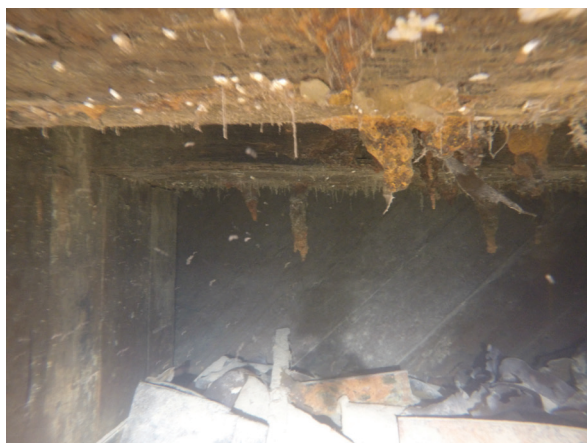
Figure 5.4.3: Interior view of the fore hold, facing the bow, showing transverse watertight bulkhead, wing bulkhead (at left) and debris and artefact accumulation (Photo: J. Moore, Parks Canada; 89Mo2777EF).
