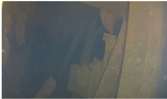
Figure 5.4.2: View into the "Carpenter's Storeroom" (Video Still: R. Harris, Parks Canada; 89M2016R003_13213).
