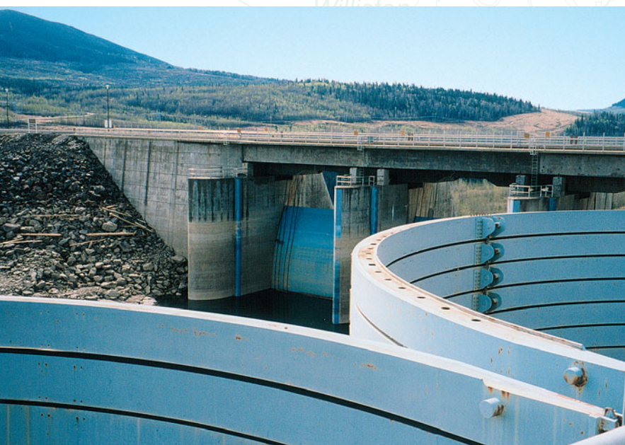
W.A.C. Bennett Dam (AENV)
