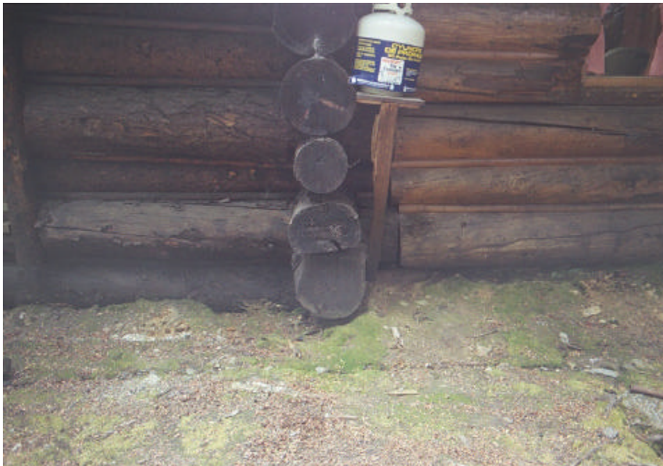
Figure 2: Units 1A and 1B before excavation. Note join in structure between the earlier log cabin and the later annex. Photograph 404T17M.
