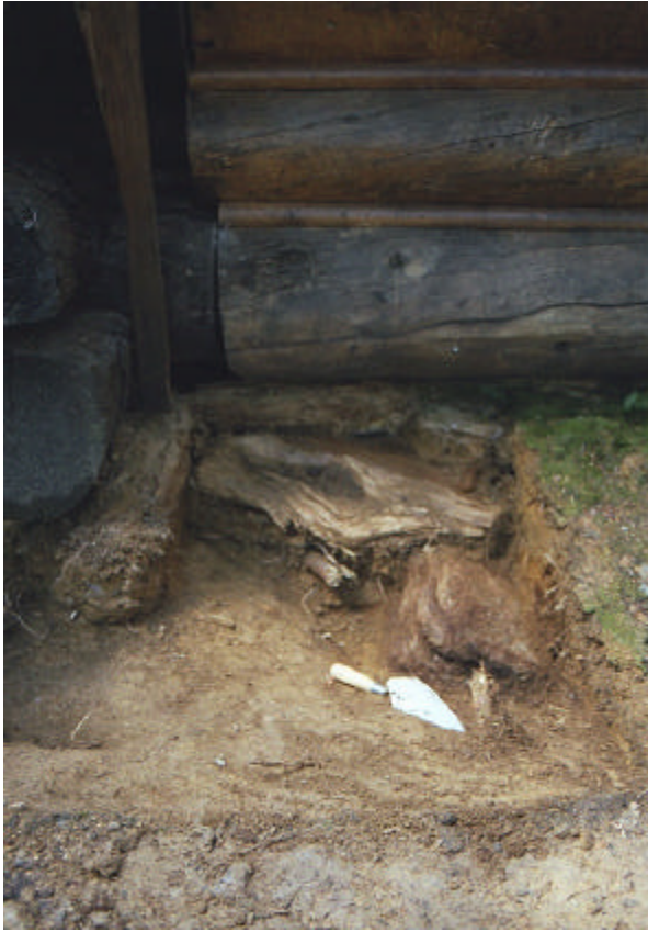
Figure 3: Post excavation photograph of excavation unit 1B. Photograph 404T20M.
