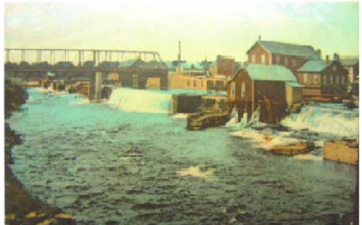
Figure10: Leggot Power House front right of the photograph Photo credit: L.H.S
