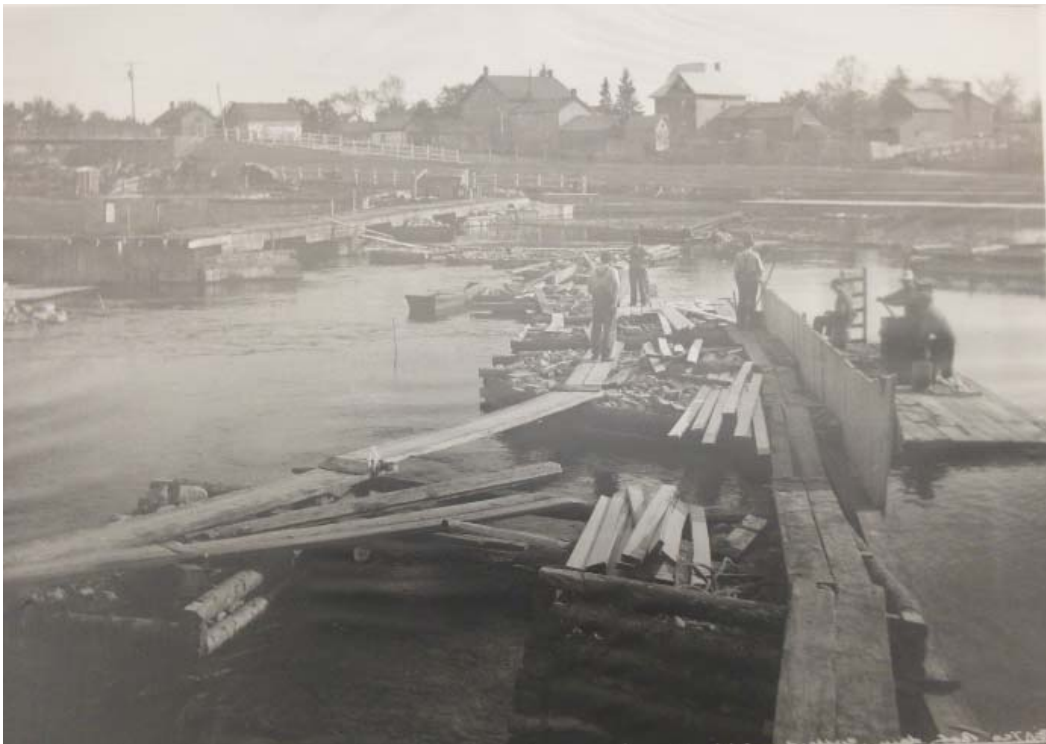
Appendix G: Construction of the dam. Lakefield Historical Society: Delladone collection
