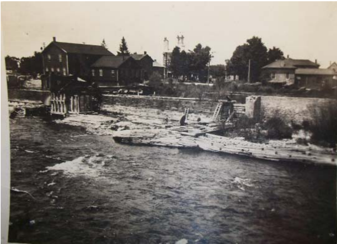
Appendix F: Wooden foundation of Woolen mill to the right. The wooden fenced in area is thought to be the ruins of Leggotts power house. Lakefield Historical Society: Delladone Collection
