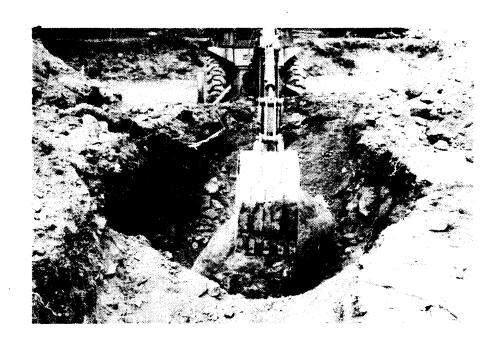
Photo 17. Boulder encountered in a house excavation in shallow gravel over till, north of Hilton lake (Twin Lakes).
