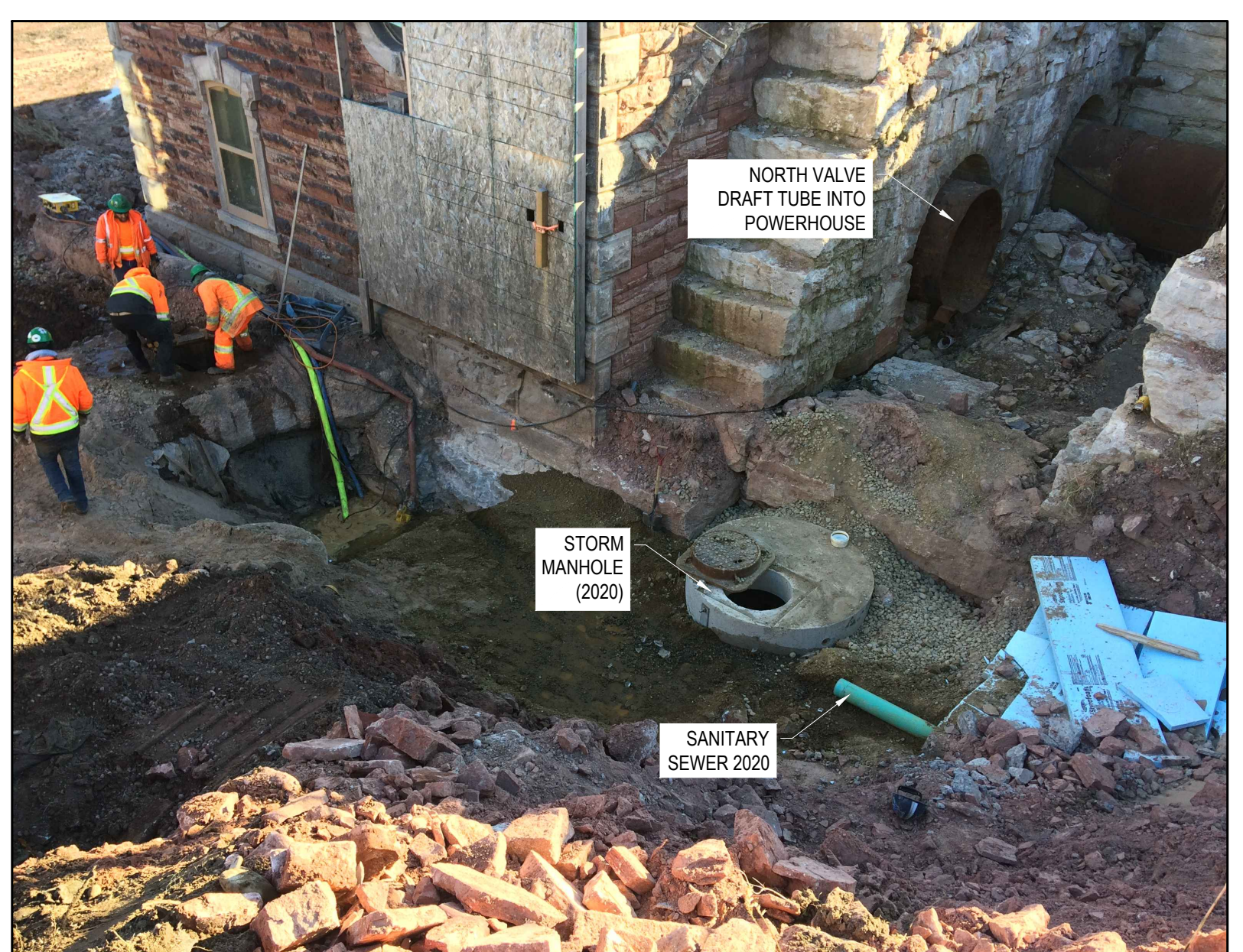
NEW STORM SEWER MANHOLE 2019 SCALE: NTS
