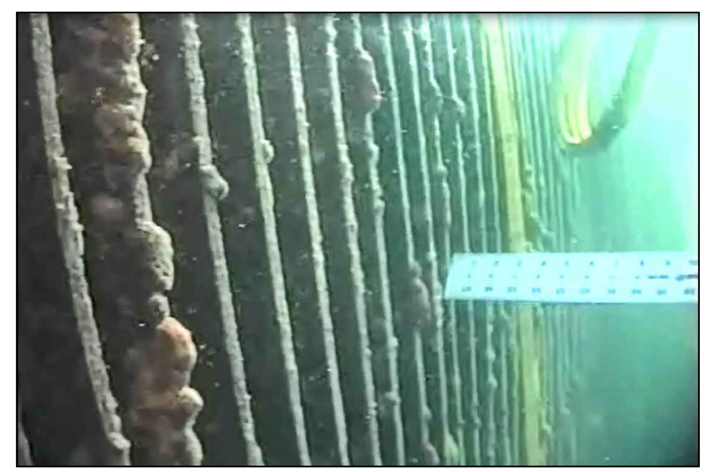
CONCAVE DEFLECTION OF INTAKE SCREEN SCALE: NTS
