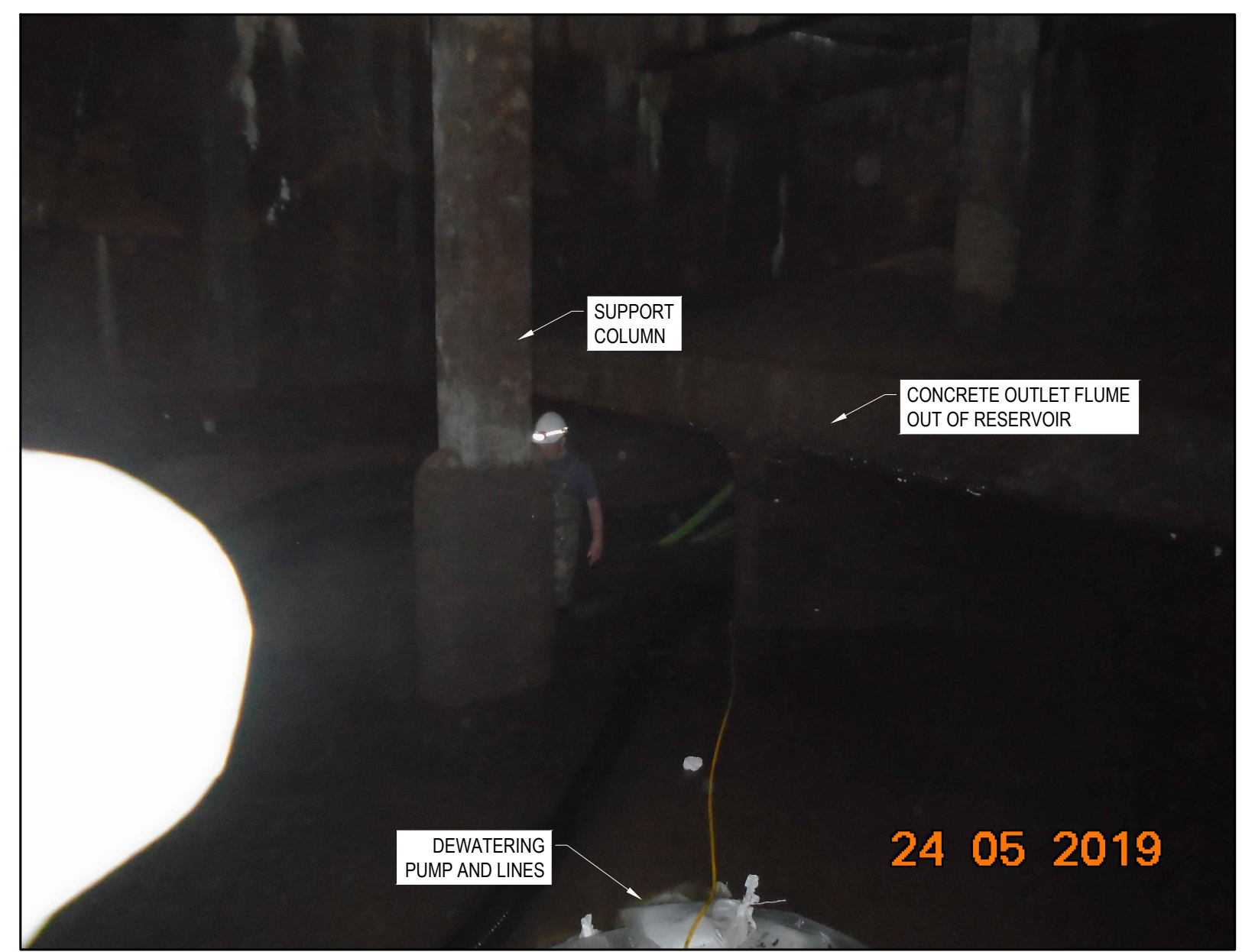
RESERVOIR OUTLET FROM WITHIN RESERVOIR SCALE: NTS
