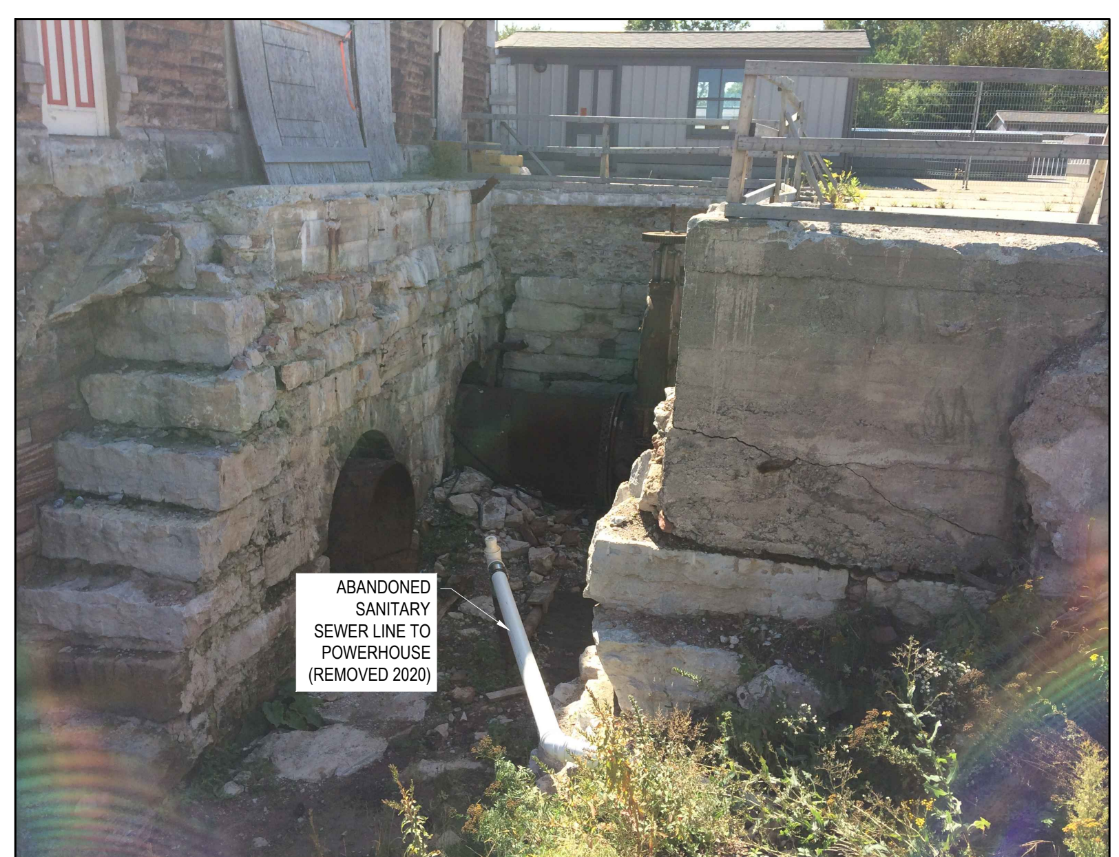
VALVE CHAMBER AT POWERHOUSE SCALE: NTS
