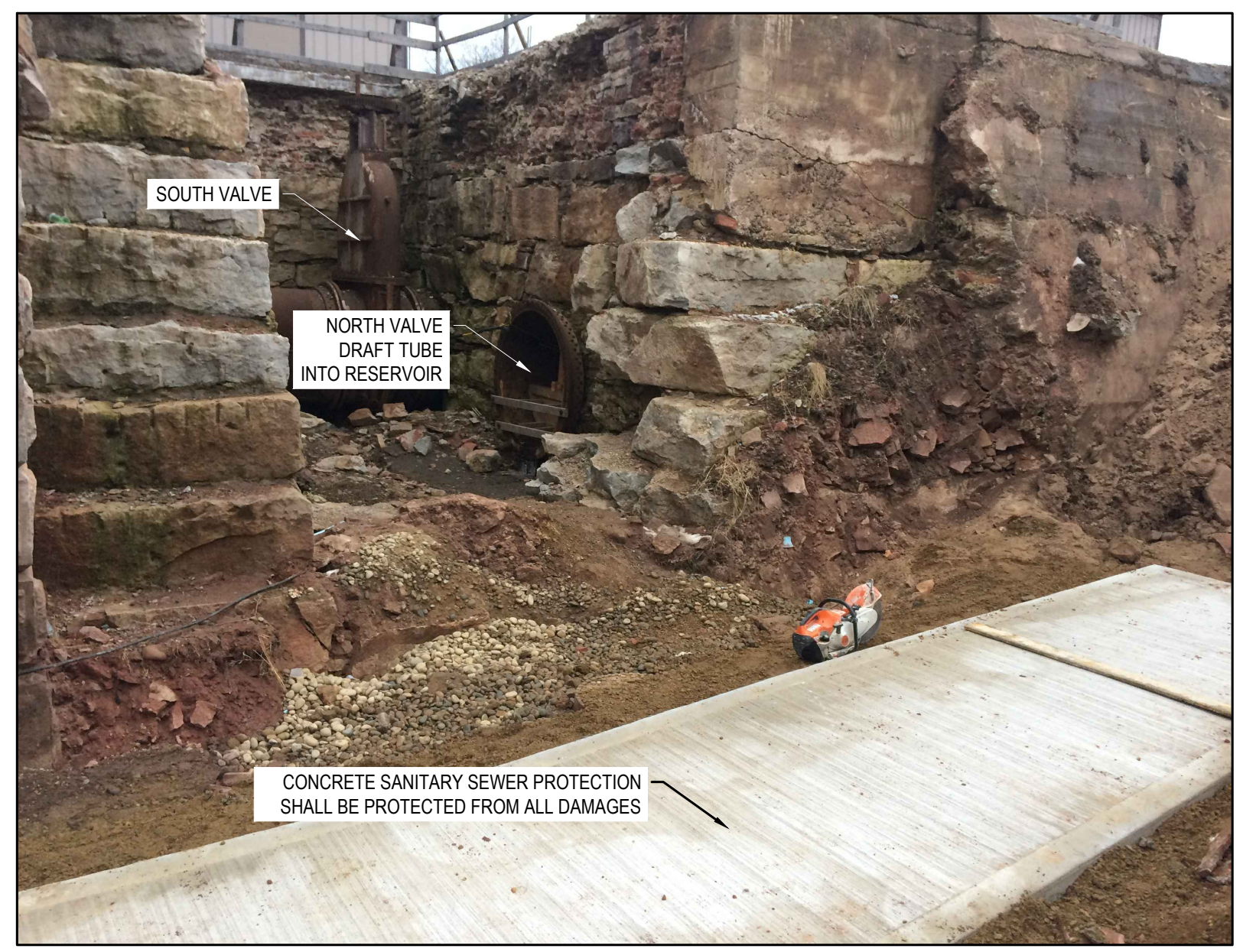
VALVE CHAMBER WITH SOUTH VALVE SCALE: NTS
