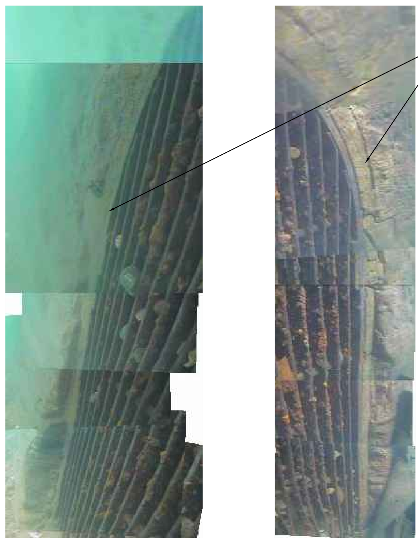
RIGHT AND LEFT SIDE JOGS OF STONE WALL AT THE INTAKE SCREEN SCALE: NTS
