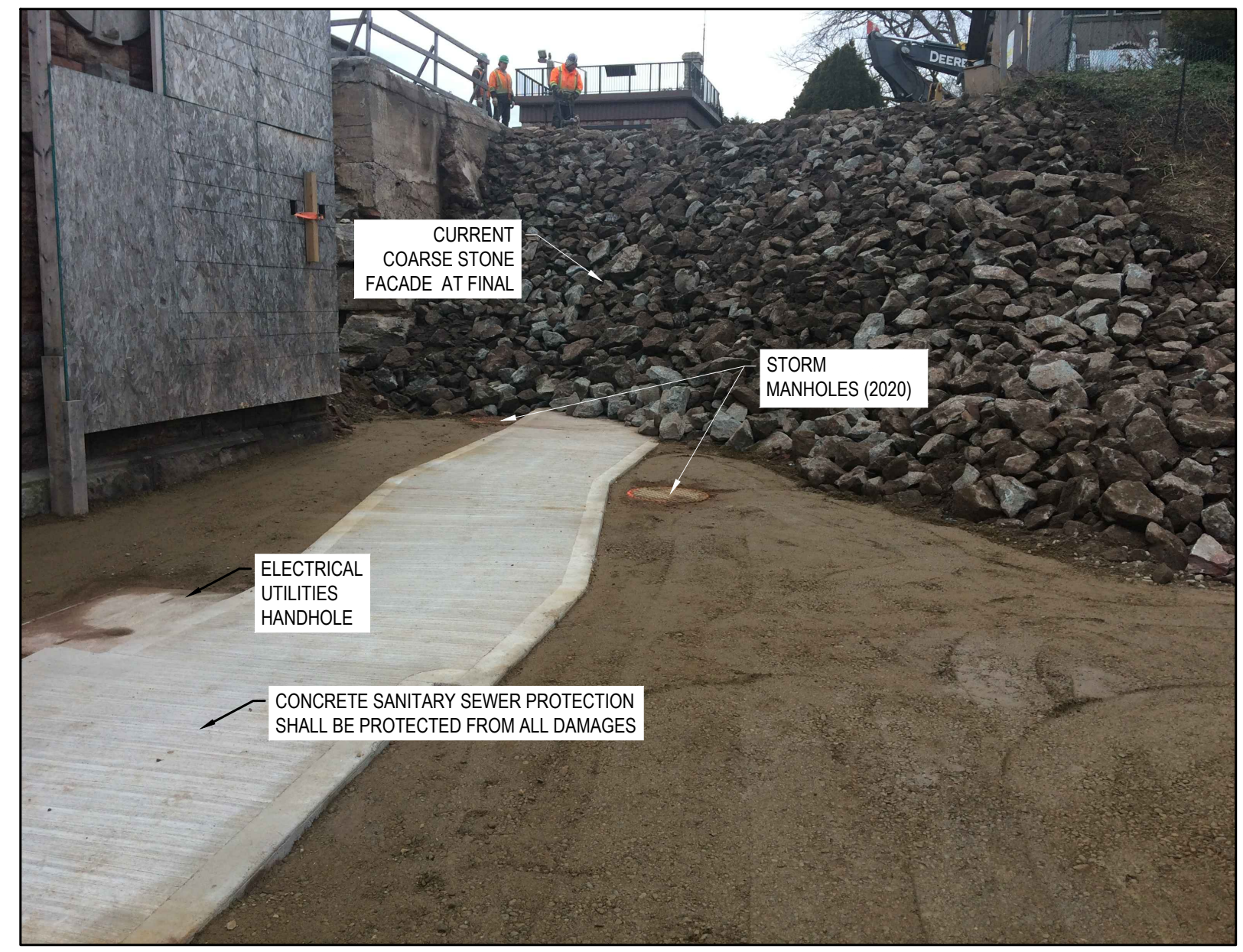
CURRENT CONDITIONS AT VALVE CHAMBER SCALE: NTS
