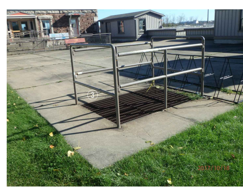
CURRENT CONDITIONS - PHOTO #3
