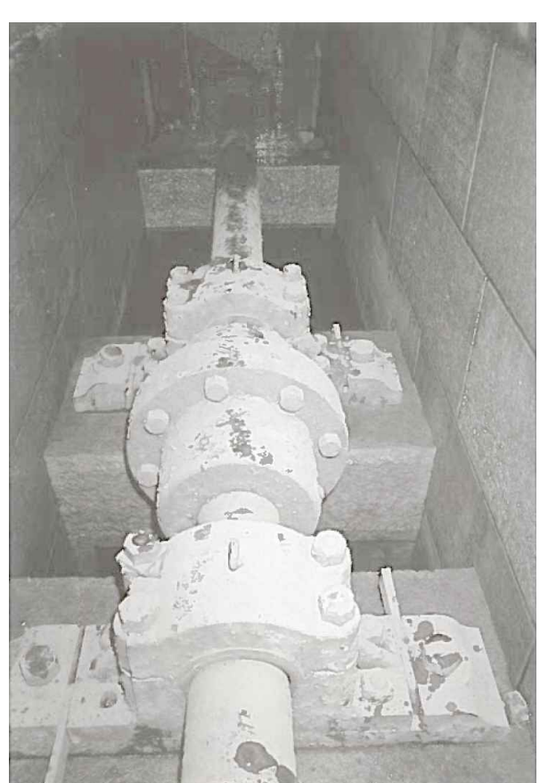
NORTH VALVE SHAFT CHAMBER SCALE: NTS (LOOKING NORTH)
