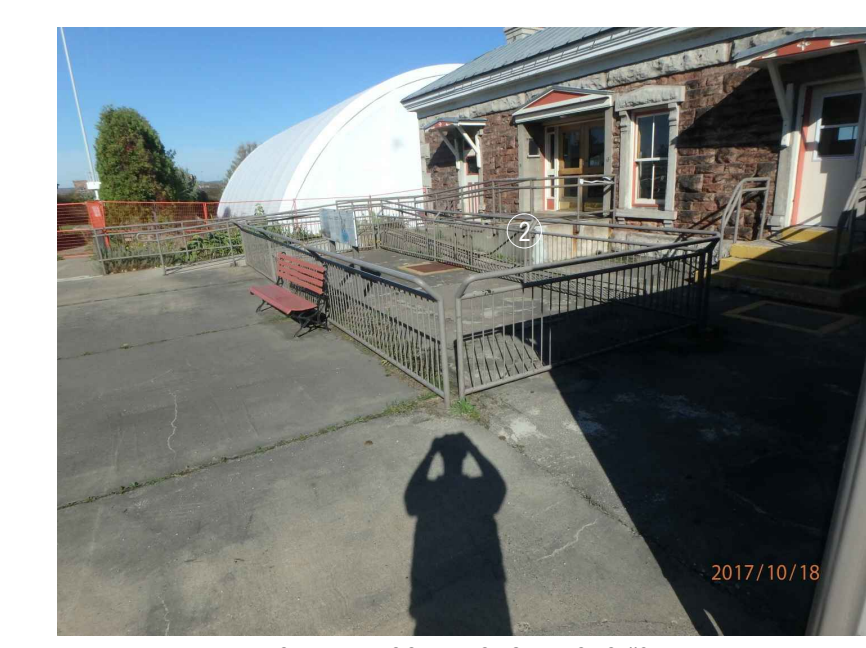
CURRENT CONDITIONS - PHOTO #2
