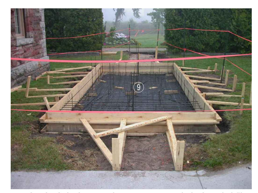
EXISTING HISTORIC VALVE MONUMENT PAD REINFORCING - PHOTO #8 (SHOWN FOR REFERENCE)
