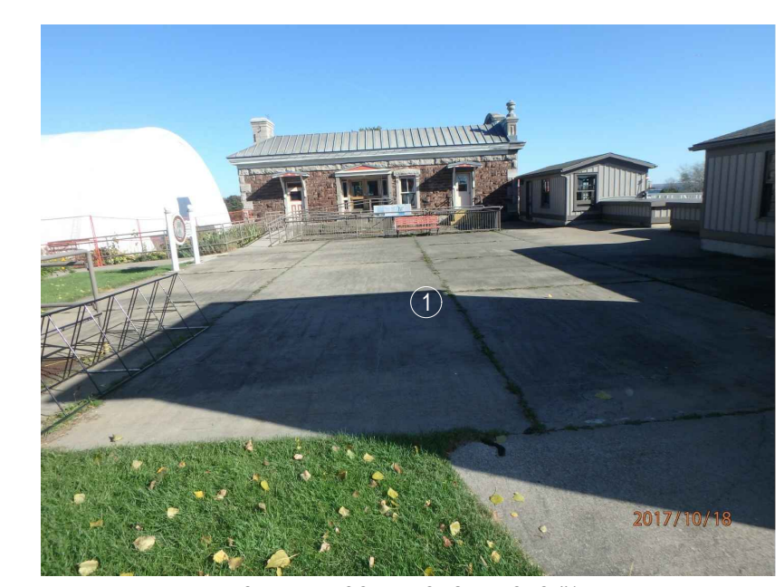
CURRENT CONDITIONS - PHOTO #1
