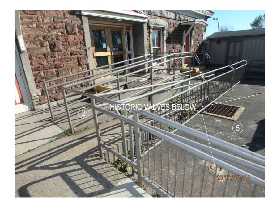
CURRENT CONDITIONS - PHOTO #5
