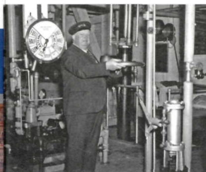
The speed and direction of the engines was controlled by the engineer as directed from the wheelhouse via the ship's telegraph, augmented by bells and a voice tube.
