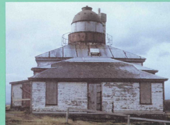
Lighthouse before restoration Le phare avant sa restauration
