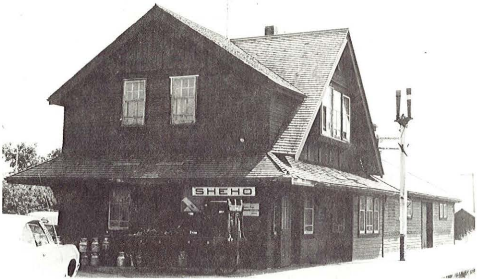
The massive appearance of the Sheho-type station is obvious. The overall effect of the front dormer with its bay, awning, and rectangular office bay makes for a striking structure. This 1971 photograph reveals that L.C.L. freight shipments were still being delivered by the CP to various Saskatchewan depots. Constructed in 1927, this building may have replaced an earlier one. (Charles W. Bohi Photo)
