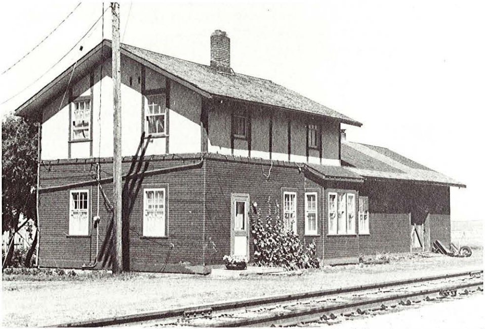
Located east of Regina on the Canadian Pacific mainline, the Balgonie depot is typical of stations originally built by the company. The lack of an overhang meant the office and bay received the full effect of the summer sun. The shade provided by even a small overhang is shown by the shadow on the freight house. Built in 1893, the CP upgraded the Balgonie station by the application of stucco on the upper storey and the addition of "Insul-brick" on the lower walls. "Insul-brick" was also widely used on CP's Soo Line affiliate to tighten uninsulated depot structures. (Charles W. Bohi Photo)
