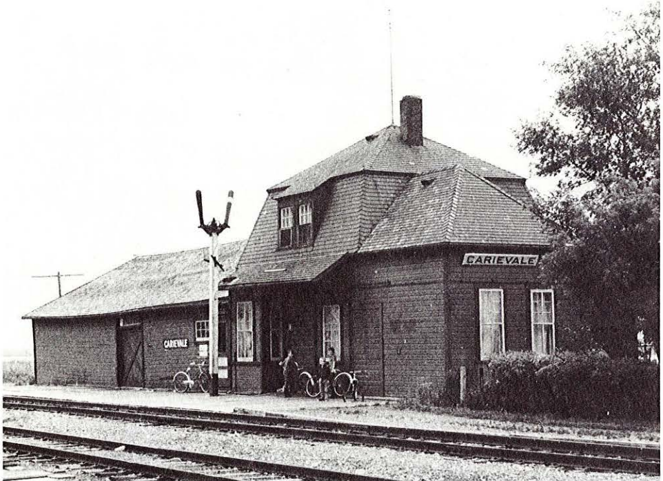
The CP opened the Carievale building in 1901. The placement of the doors at the front indicates that the waiting room was located between the office and freight house. The hip-roof addition on what would be normally the waiting-room end was almost certainly used for living space. Even in 1969, when this photograph was taken, children were still growing up in country depots. (Charles W. Bohi Photo)
