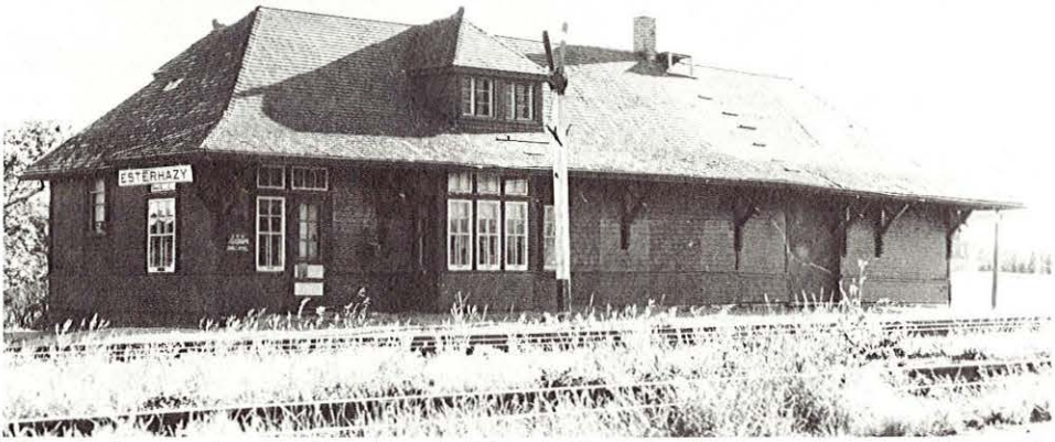
The shadows cast on the Esterhazy building indicate the shade overhangs could provide. This station has had some of its windows and doors removed over the years. Standardized plans usually were made so that they could allow easy alteration should local needs require change. (Charles W. Bohi Photo)
