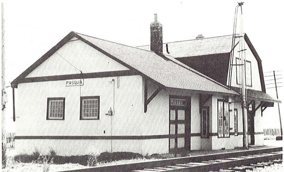
Located near Moose Jaw, the Pasqua station is an earlier example of the Sinaluta-style depot. Built in 1903 at the junction of the mainline and an important branch to North Portal, this building is one of the very few CP stations in Saskatchewan that had stucco applied. (Charles W. Bohi Photo)
