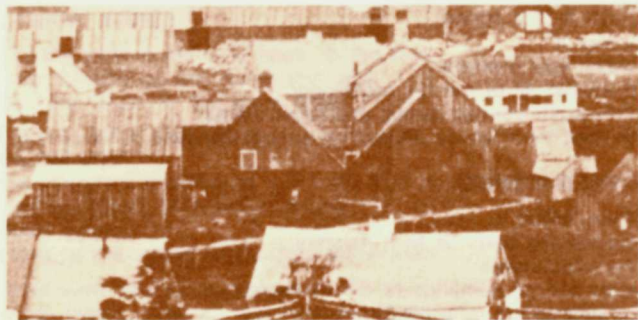
Blast-furnace, 1880 Section of photograph Eric Sprenger Collection Montreal, Canada.
