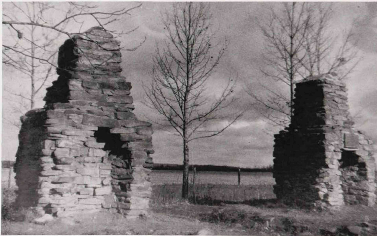
All that remains of Rocky Mountain House—the chimneys of the main building in the 1864 fort.
