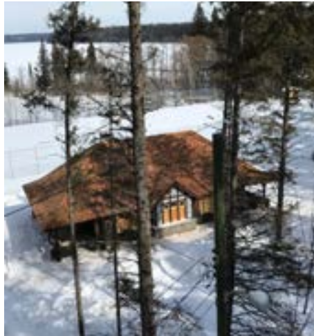
Newly re-shingled Tennis Clubhouse
