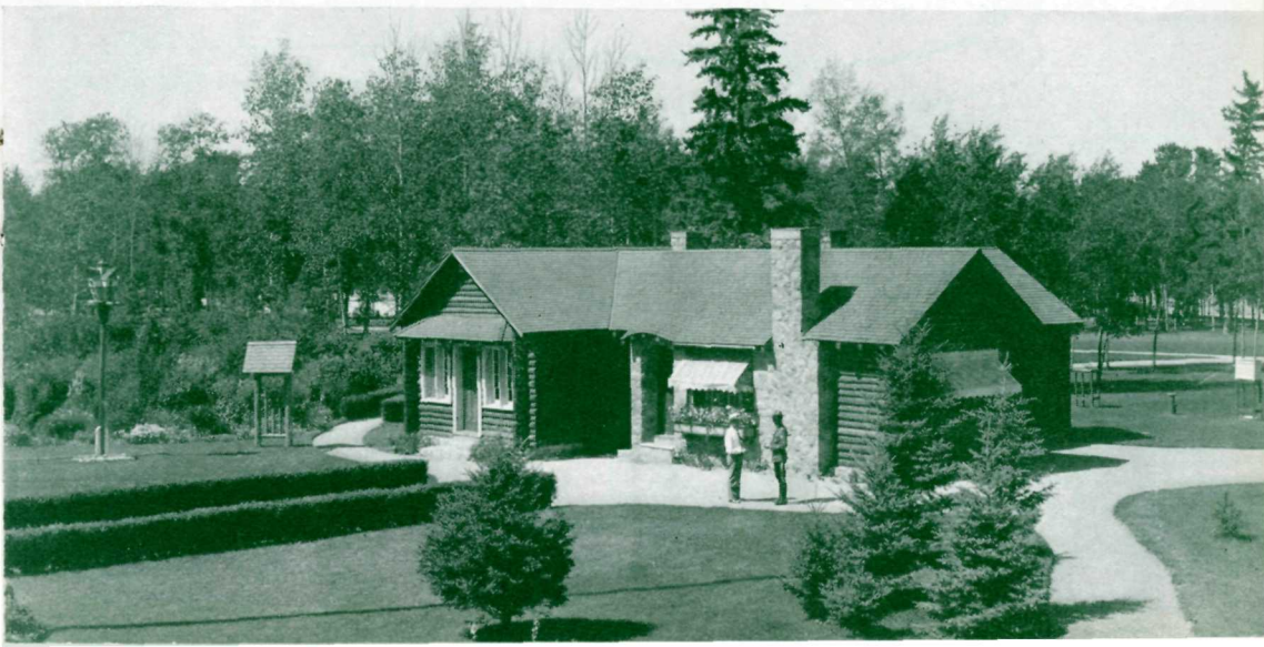
The Administration Building
