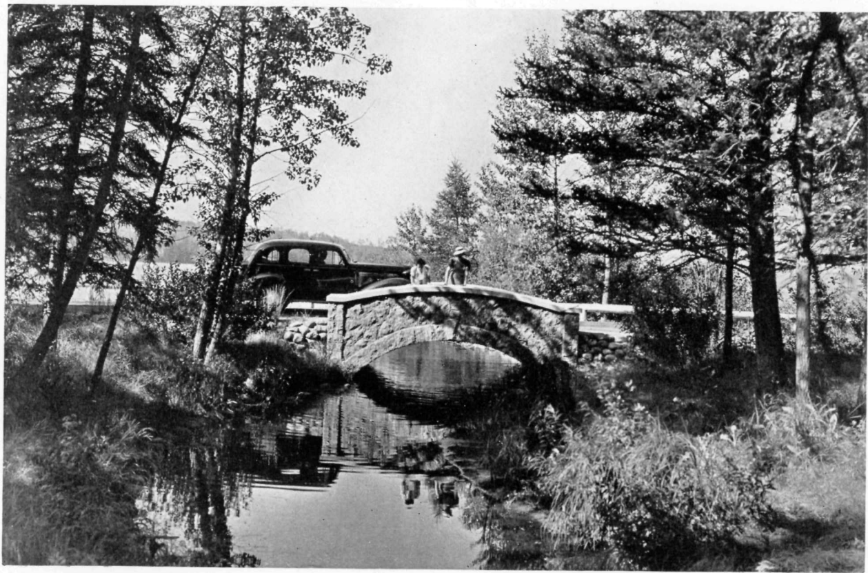
Bogey Creek Bridge on the Glen Beag Drive, Riding Mountain National Park
