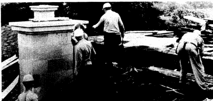
Workmen removing asphalt shingles from roof prior to laying of new slate roof. Note re-constructed stone chimney above roof. (Parks Canada, 1981)
