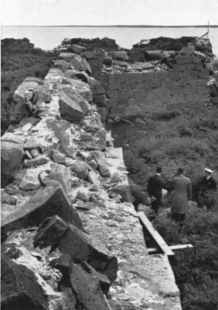
In 1934, the year before the fort was repaired, Governor Cooper (centre) visited the ruins with Michael Lubbock and Capt. Smellie. Note the absence of mortar between the stones.
