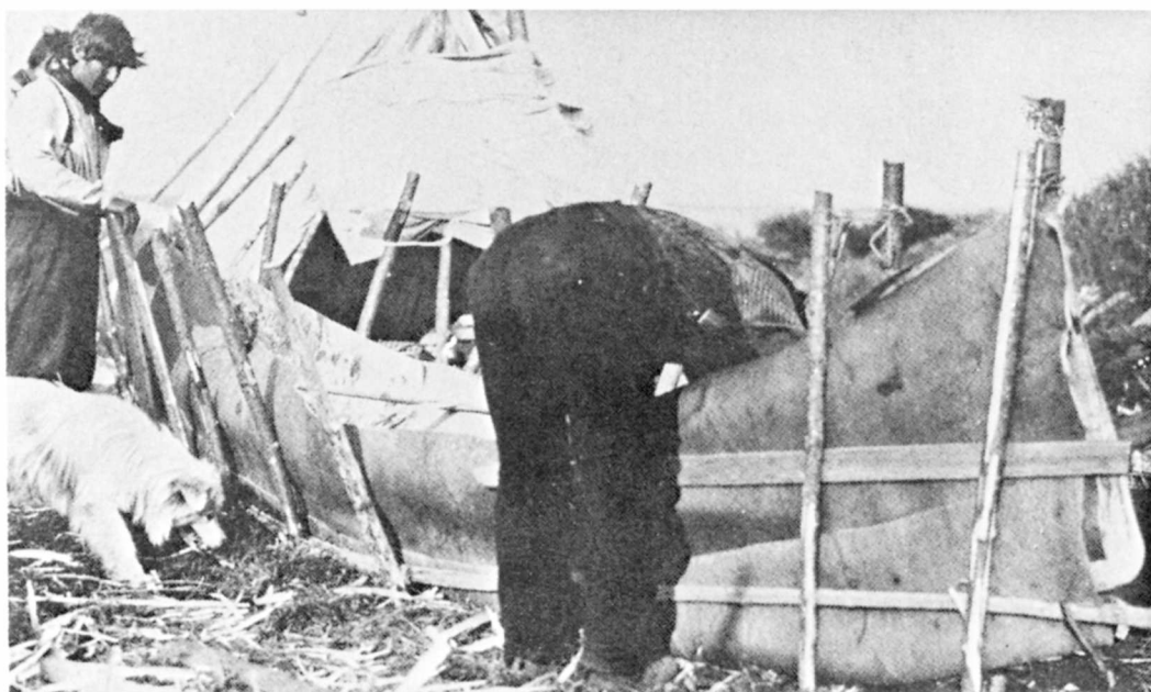
40 Assembling a birch bark canoe (courtesy Geological Survey of Canada)
