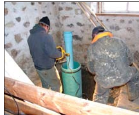
INSTALLATION OF WATER MAIN, STONE HOUSE PARKS CANADA / S. HELFRICK / 2008
