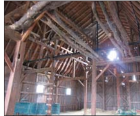
FIRE SUPPRESSION SYSTEM IN BARN LOFT PARKS CANADA / C. ARCHER / 2009
