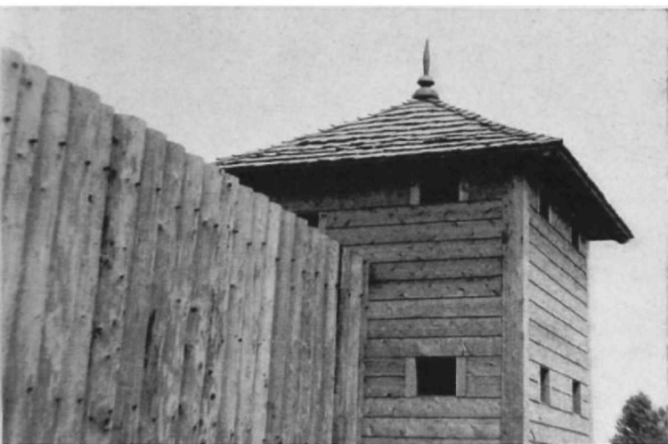
The rebuilt northeast bastion with part of the outside of the palisade.
