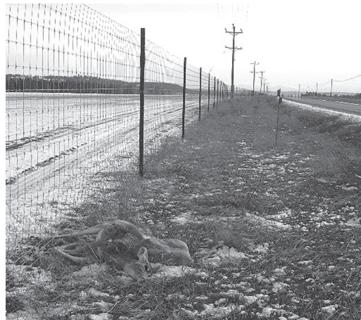
Figure 9. Fences generally exclude animals from entering the roadway, but occasionally they become trapped in the narrow corridor and cannot escape because of fences. One-way gates are possible options to allow passage of animals from the roadside to the safe side. Highway 93/95 near Skookumchuk Prairie, Wasa, BC. 8 March 2003 (Larry Halverson).
