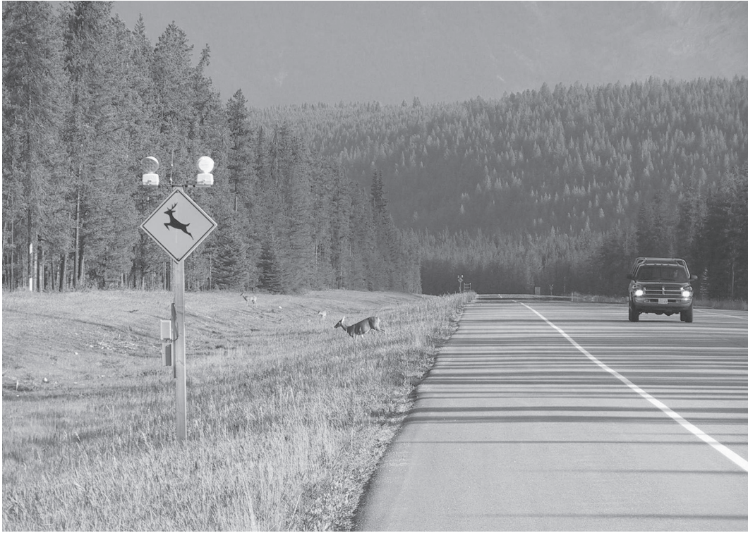
Figure 10. The Wildlife Protection System uses an infrared camera to detect animal presence along roadways, which subsequently triggers flashing lights warning approaching motorists. Highway 93 near Dolly Varden Creek, Kootenay National Park, BC. (Alan Dibb).
