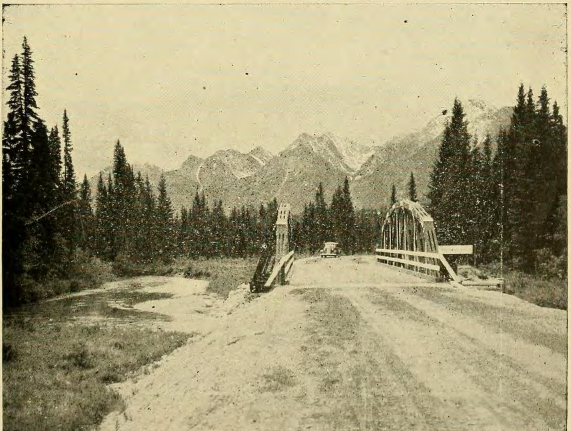
Bridge at Kootenay River Crossing, Kootenay National Park, B. C.
