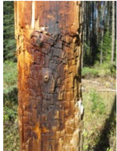
Figure29. These images of two heavily oiled power line poles in YNP, show extensive damage by bear bites and scratches. That various petroleum products are attractants to bears is undisputed and lends credence to the suggestion that the metabolic effects on bears should be investigated. (Photo courtesy of Ken Schroeder, YNP)
