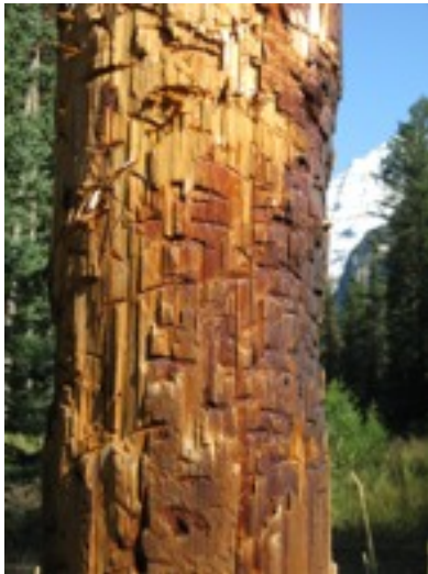
Figure29. These images of two heavily oiled power line poles in YNP, show extensive damage by bear bites and scratches. That various petroleum products are attractants to bears is undisputed and lends credence to the suggestion that the metabolic effects on bears should be investigated. (Photo courtesy of Ken Schroeder, YNP)
