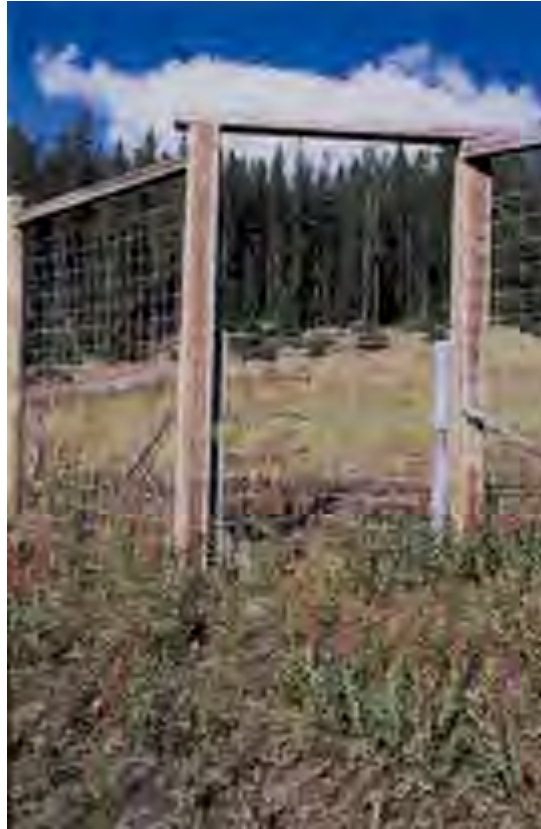
Figure 45: One-way elk gate in British Columbia, (© Marcel Huijser).
