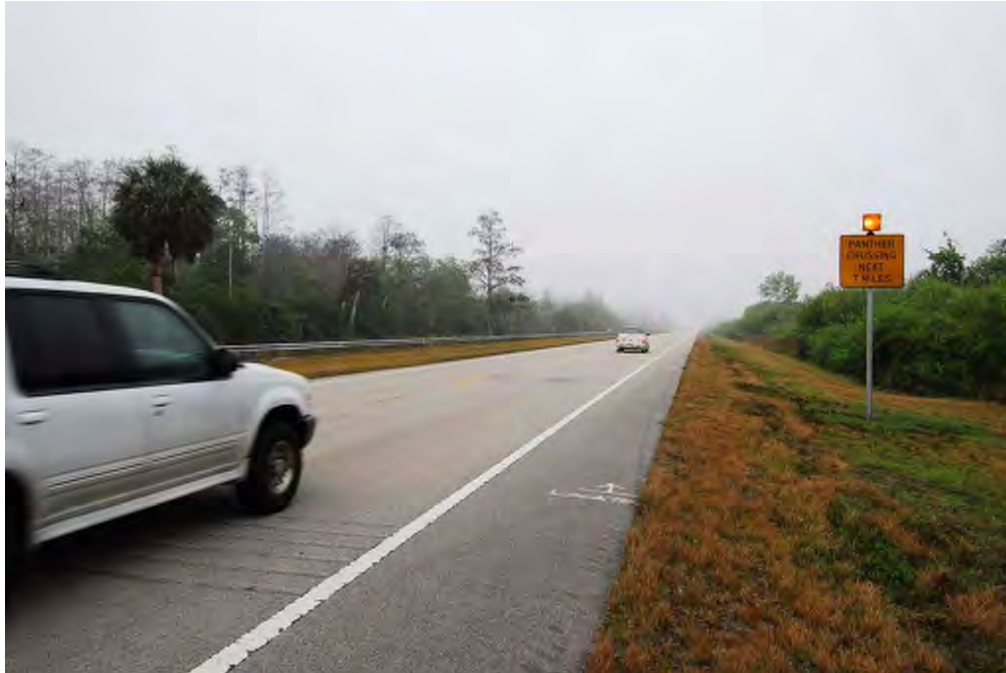
Figure 3: Patches of rumble strips accompany a panther warning sign along State Route 29 in southern Florida (© Marcel Huijser).
