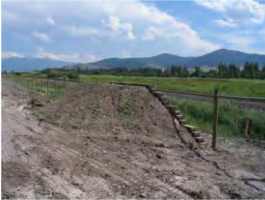
Figure 42: A jump-out along a 2.4 m (8 ft) high fence along U.S. Highway 93 in Montana (© Marcel Huijser).
