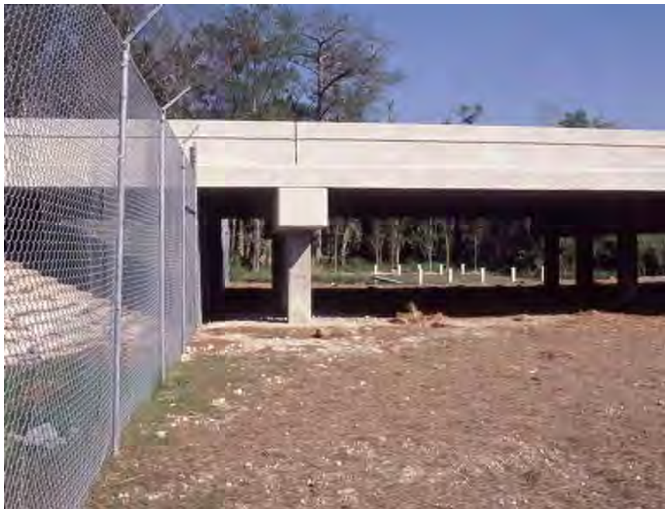
Figure 55: Underpass in southern Florida that allows for ecosystem processes (hydrology) as well as wildlife use, including the Florida Panther (© Marcel Huijser).
