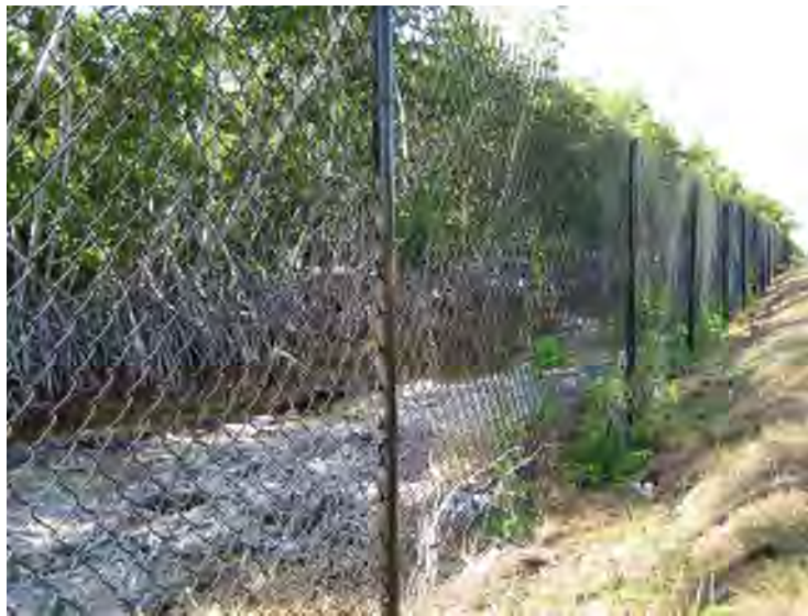
Figure 36: A 1.83 m (6 ft) high chain link fence along U.S. Hwy 1 between Florida City and Key Largo, Florida, has been coated with plastic to make the fence blend in with its surroundings (© Marcel Huijser).
