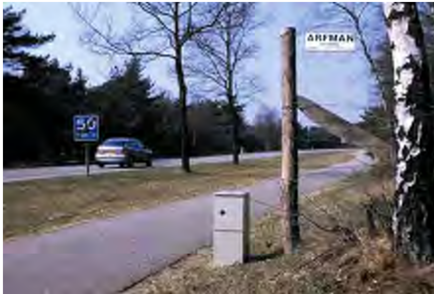
Figure 40: Gap in a wildlife fence combined with an animal detection system, wildlife warning signs and advisory speed limit reduction, the Netherlands (© Marcel Huijser).
