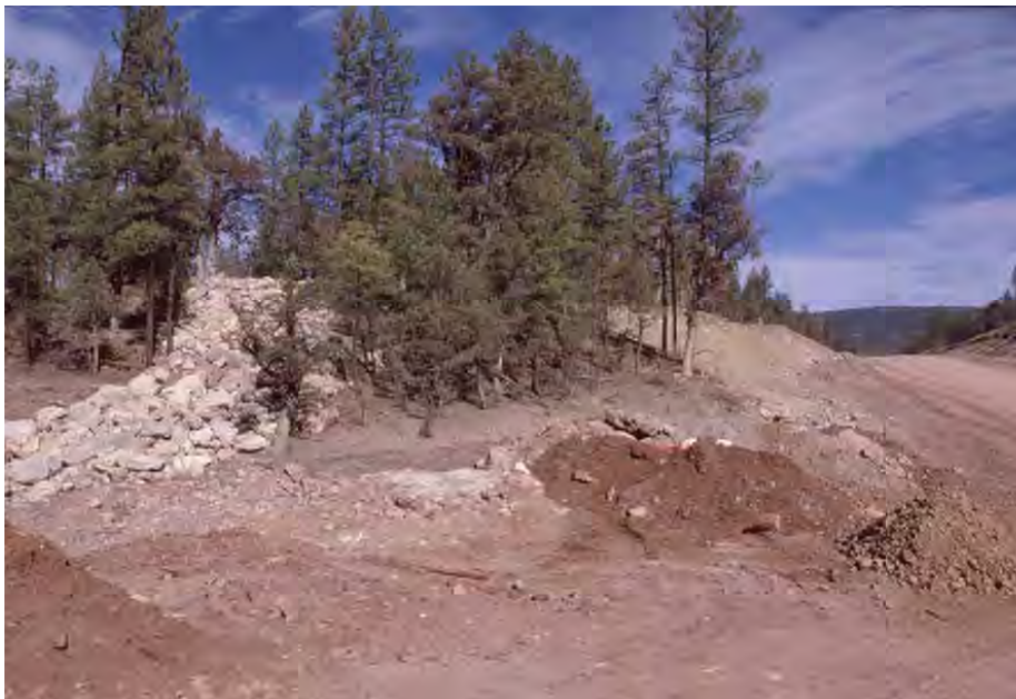
Figure 38: Large boulders placed in the right-of-way as a barrier to elk and deer with a view of State Route 260 (under construction) in Arizona (© Marcel Huijser).
