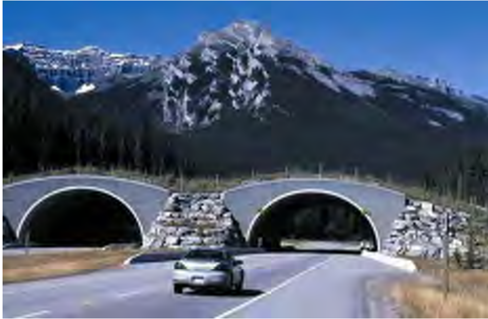
Figure 50: Wildlife overpass along the Trans-Canada Highway in Banff National Park, Alberta (© Marcel Huijser).
