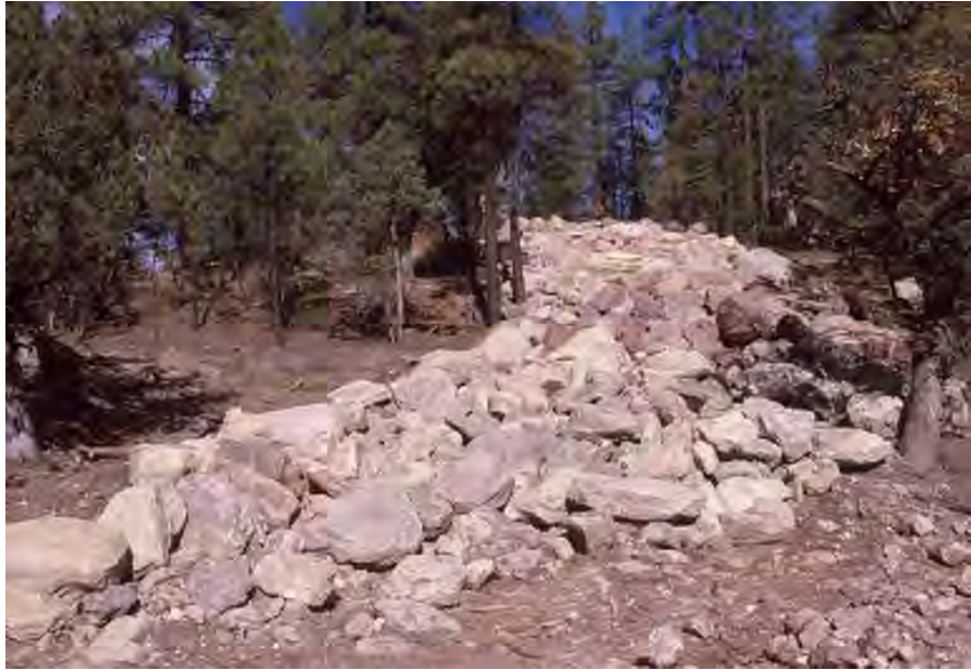
Figure 37: Large boulders placed in the right-of-way as a barrier to elk and deer along State Route 260 in Arizona (© Marcel Huijser).
