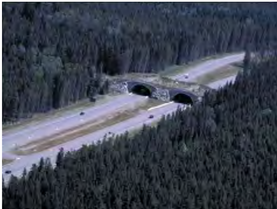
Figure 51: Red Earth Overpass on the Trans-Canada Highway (©Tony Clevenger).
