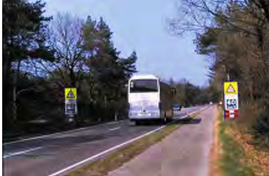
Figure 39: Gap in a wildlife fence accompanied by wildlife warning signs and advisory speed limit reduction, the Netherlands (© Marcel Huijser).
