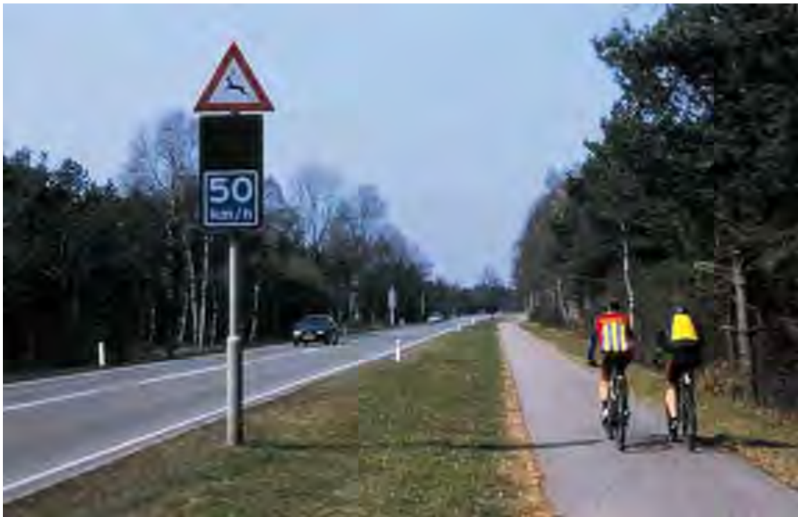
Figure 4: Advisory speed limits accompany a deer warning sign near ‘t Harde, The Netherlands (© Marcel Huijser). Note: The LED part of the warning sign is linked to an animal detection system, but the advisory speed limit reduction sign is always visible in daylight, regardless of the presence and detection of large animals.
