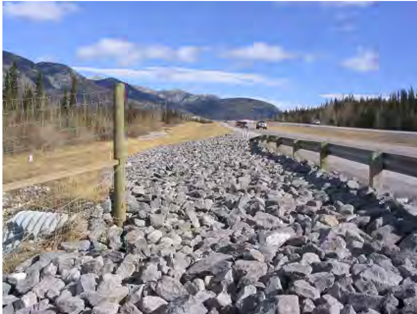
Figure 41: The boulder field at the fence end at Dead Man's Flats along the Trans-Canada Highway east of Canmore, Alberta (© Bruce Leeson).
