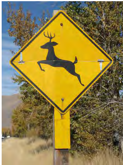
Figure 17: A permanent deer warning sign in Idaho has hinges, allowing for its seasonal use (© Marcel Huijser).
