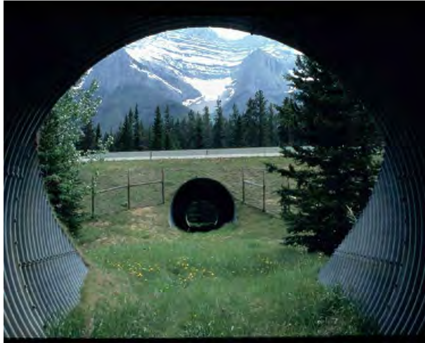
Figure 52: A large wildlife crossing culvert along the Trans-Canada Highway in Banff National Park, Alberta (© Tony Clevenger).
