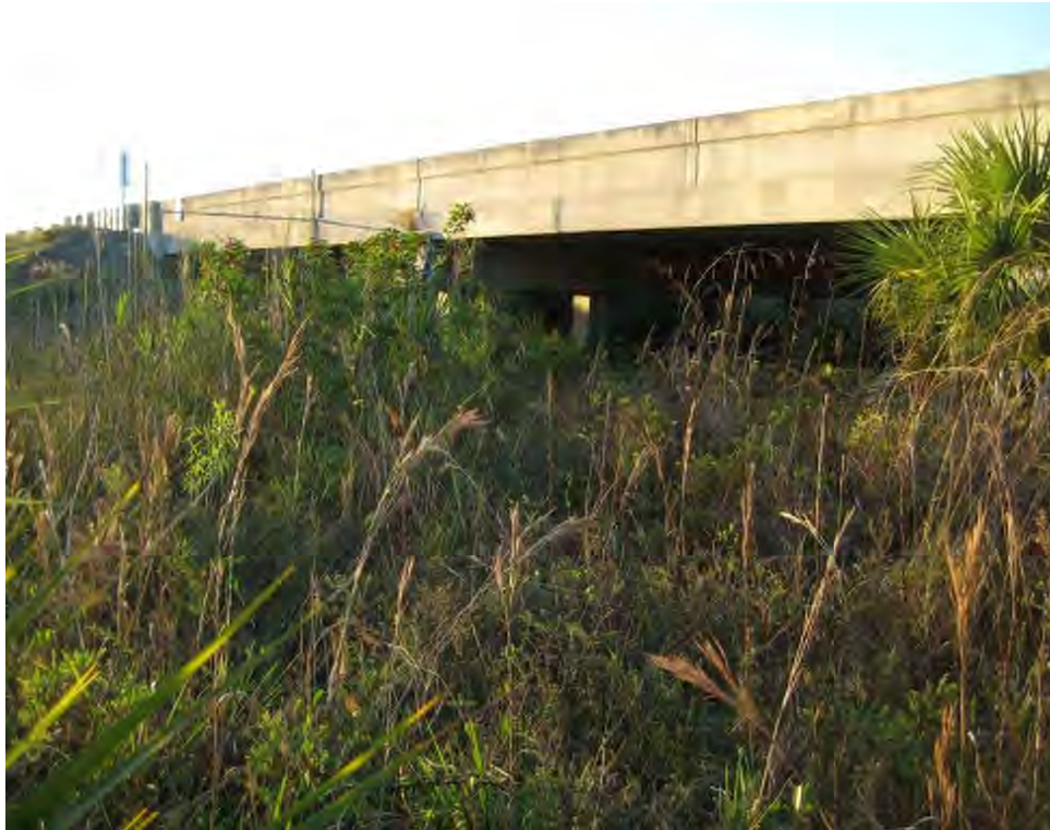
Figure 56: Underpass in southern Florida that allows for ecosystem processes (hydrology) as well as wildlife use, including the Florida Panther. Note the vegetation that provides cover (© Marcel Huijser).
