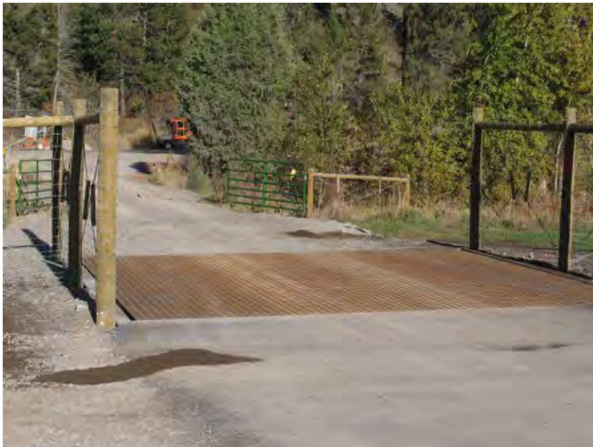
Figure 48: Wildlife guard along U.S. Highway 93 on the Flathead Indian Reservation, Montana (© Marcel Huijser).
