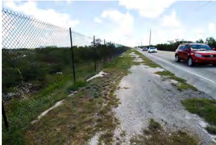
Figure 35: A 2.44 m (8 ft) high chain link fence along U.S. Hwy 1 on Big Pine Key, Florida, has been coated with plastic to make the fence blend in with its surroundings (© Marcel Huijser).
