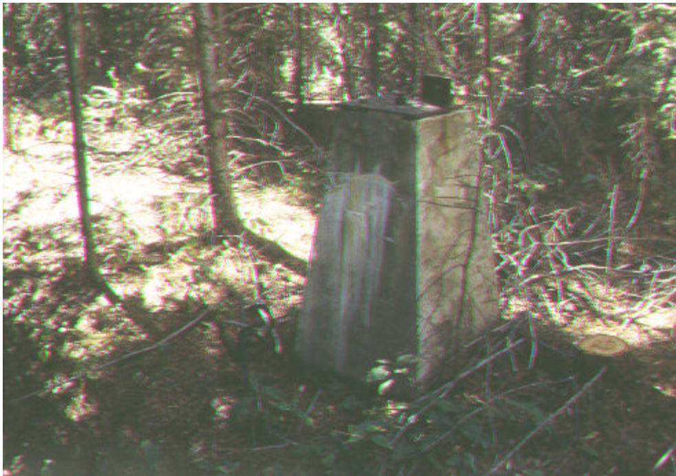
Figure 7 Concrete base of the former fire lookout tower, Mount Daer, Kootenay National Park (1473T-10t).
