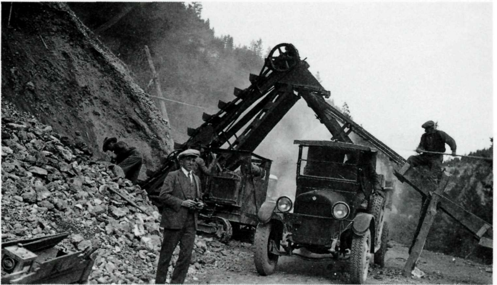
Building the Banff-Windermere Highway
