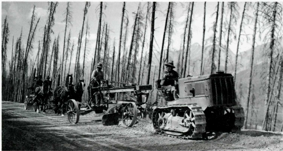
Building the Banff-Windermere Highway
