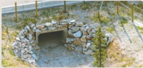
A wildlife underpass and fencing on Highway 93 South.
