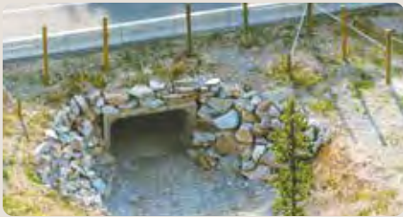
A wildlife underpass and fencing on Highway 93 south.
