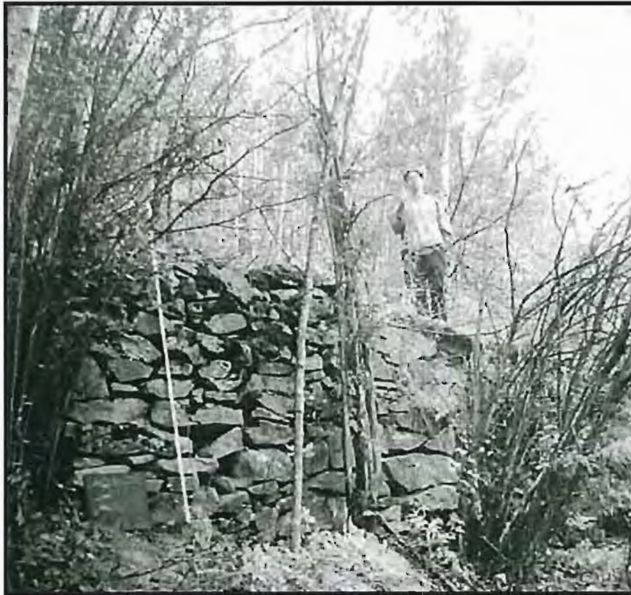
Figure 4. Large stone retaining wall at front of Crocus Bluff Platform.
