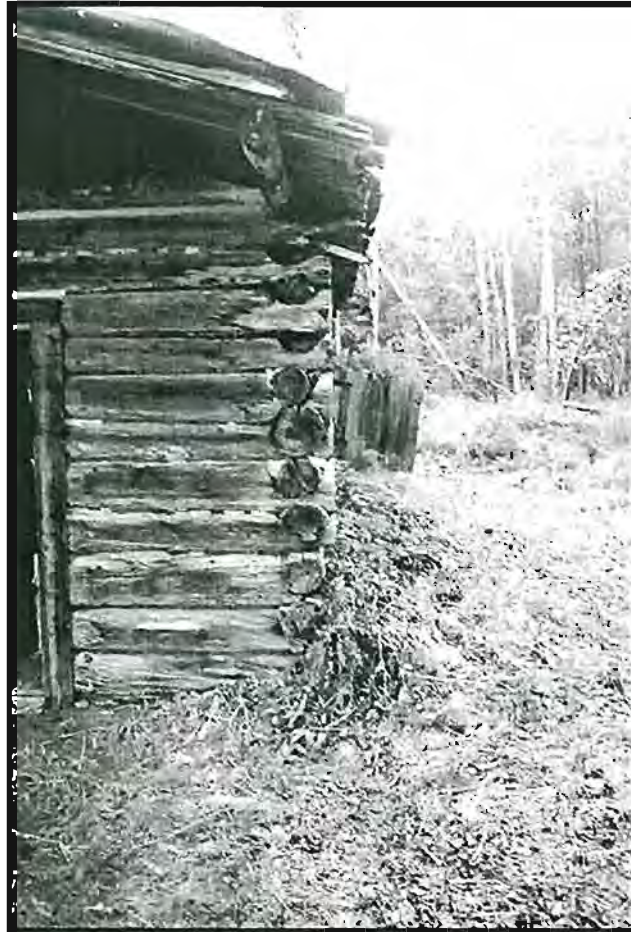
Figure 24. Log cabin located at the site of Forty Mile (LcVn-2), showing dirt mounded up against the first three courses of logs.
