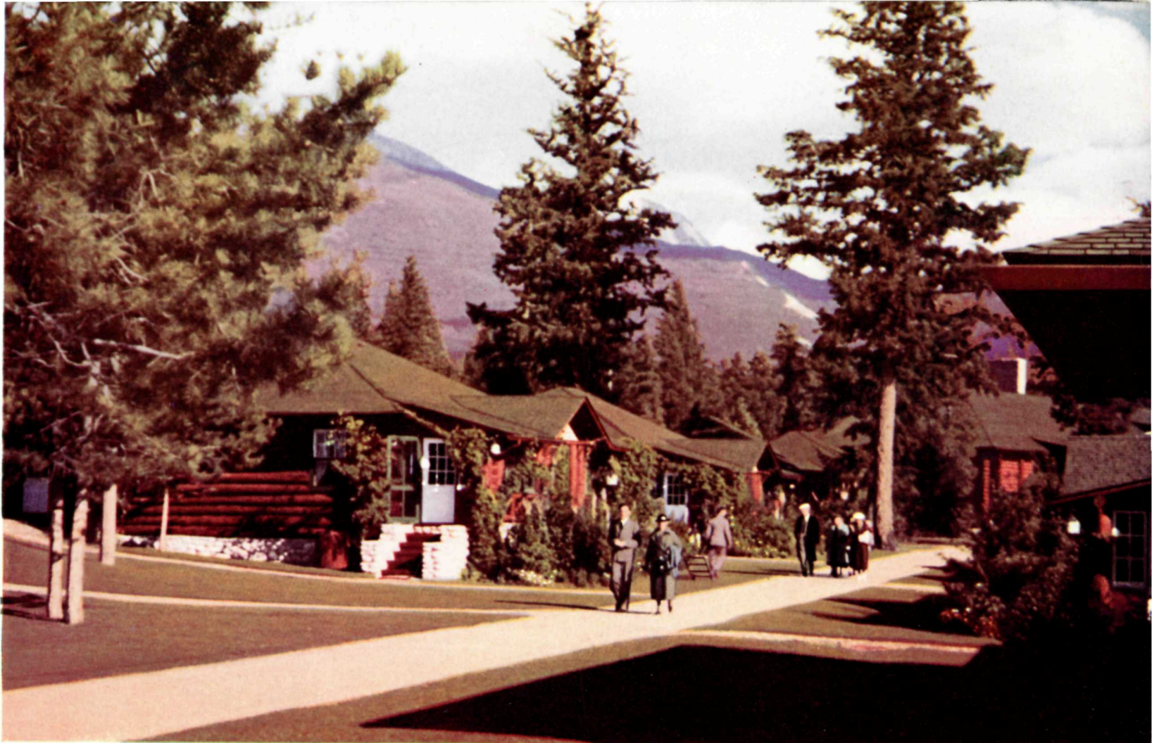
An avenue of charming Alpine lodges with landscaped foreground—Jasper Park Lodge.
