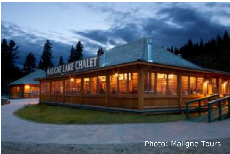
Maligne Lake Chalet, following restoration work
