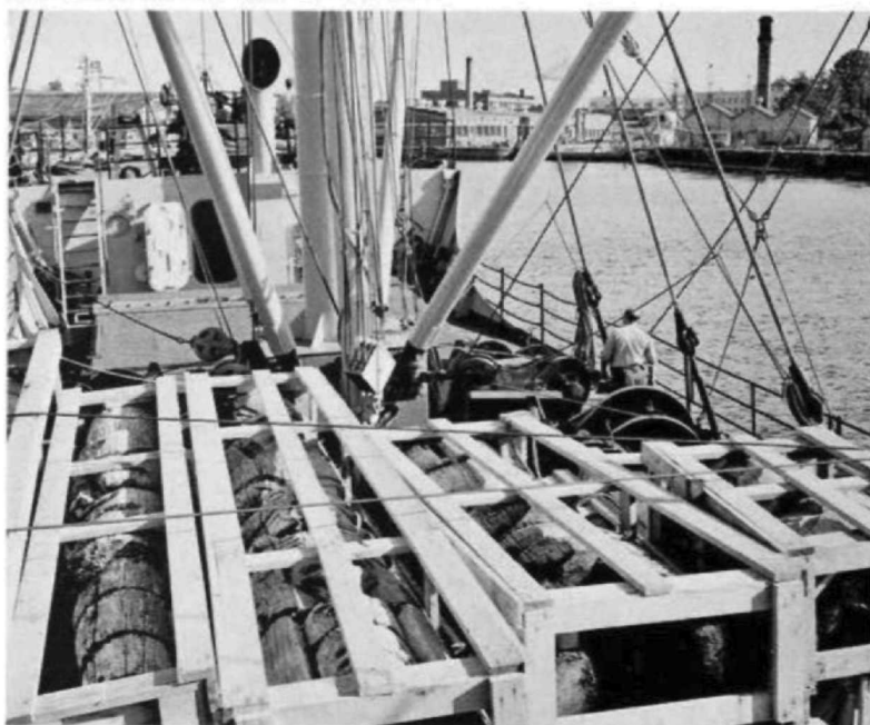
The 'Laymore' with her cargo of totem poles arrives at HMC dockyard, Esquimalt, Victoria.
