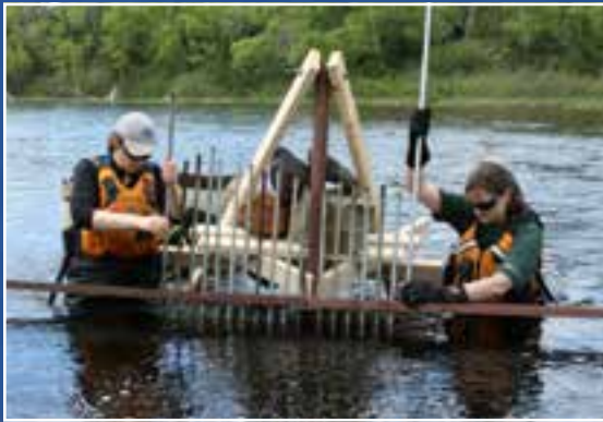
Resource Conservation staff constructing a fish fence.
