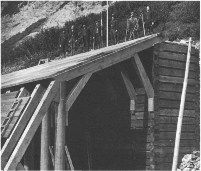
Snowshed construction along the original CPR line in Rogers Pass
