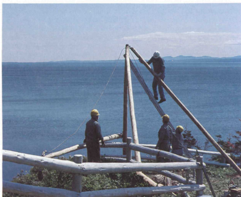
Reconstruction of a tackle with capstan
