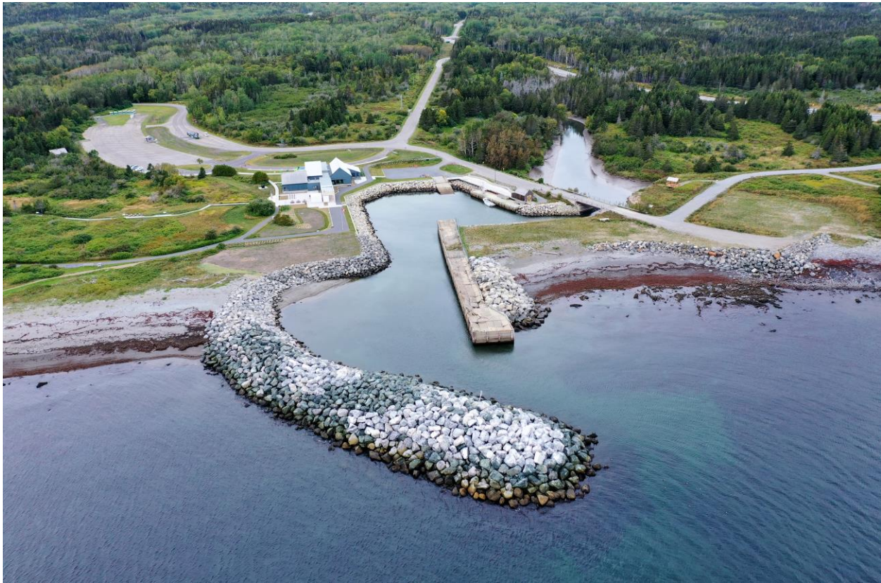
Figure 11. The Cap-des-Rosiers harbour with its restored south pier and the new Visitor Information and Discovery Centre (Jean-David Dupuis, Parks Canada).
