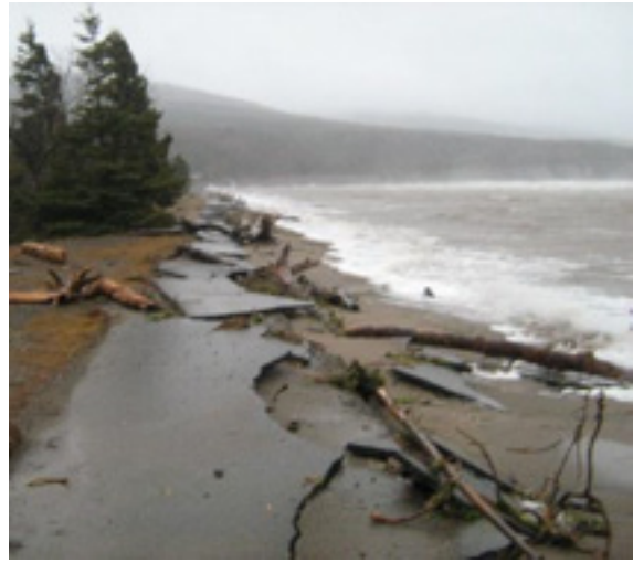
In 2016, the road was damaged again. It was rebuilt further inland, on stilts, in wood to allow it to withstand storm surges and flooding.
