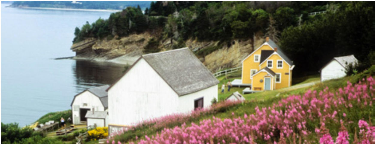
Like many sites in Forillon Park considered as cultural resources, the Blanchette homestead is located on a steep slope, vulnerable to the effects of heavy rainfall and surface run-off.
