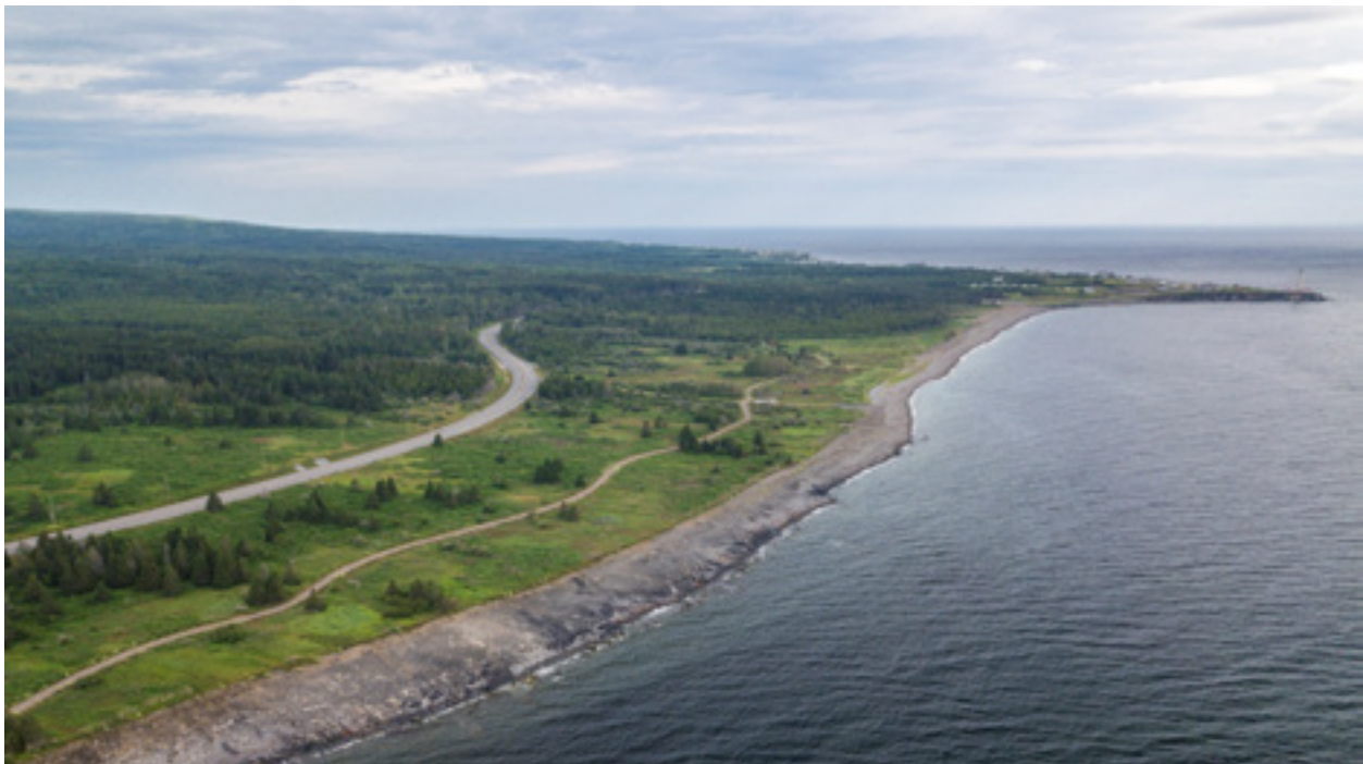
The shoreline between Cap-des-Rosiers (seen at the far right) and Cap-Bon-Ami is particularly vulnerable to storms from the northeast.
