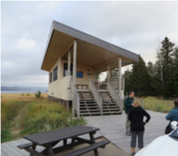
The new buildings were also built on piles further from the shore to allow them to withstand storm surges and floods.
