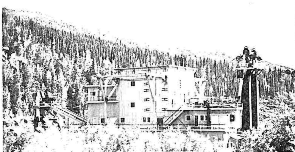
4 Dredge No. 4; port side view. (EC-CPS, KNHS, 1987.)
