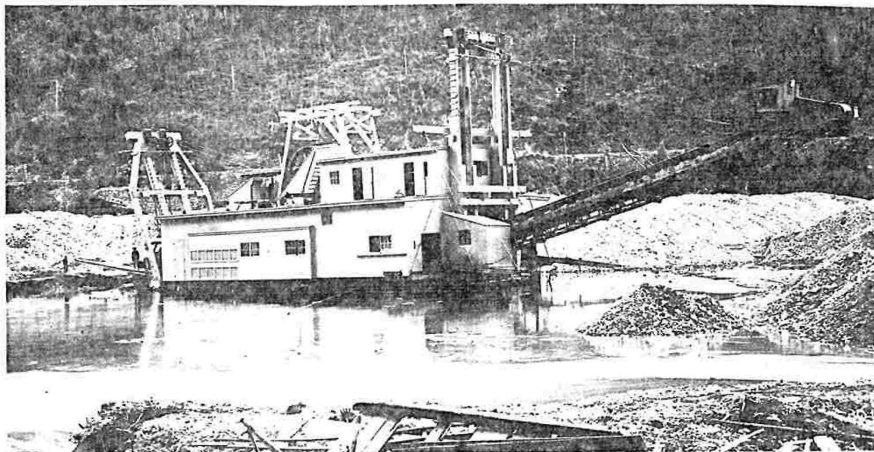
23 "Side view of Yukon Gold Co.'s Dredge No. 6 digging on Bonanza Creek, July 1908"; dredge designed by Bucyrus [Bucyrus, Ohio]. (NA/AN, C-20060.)
