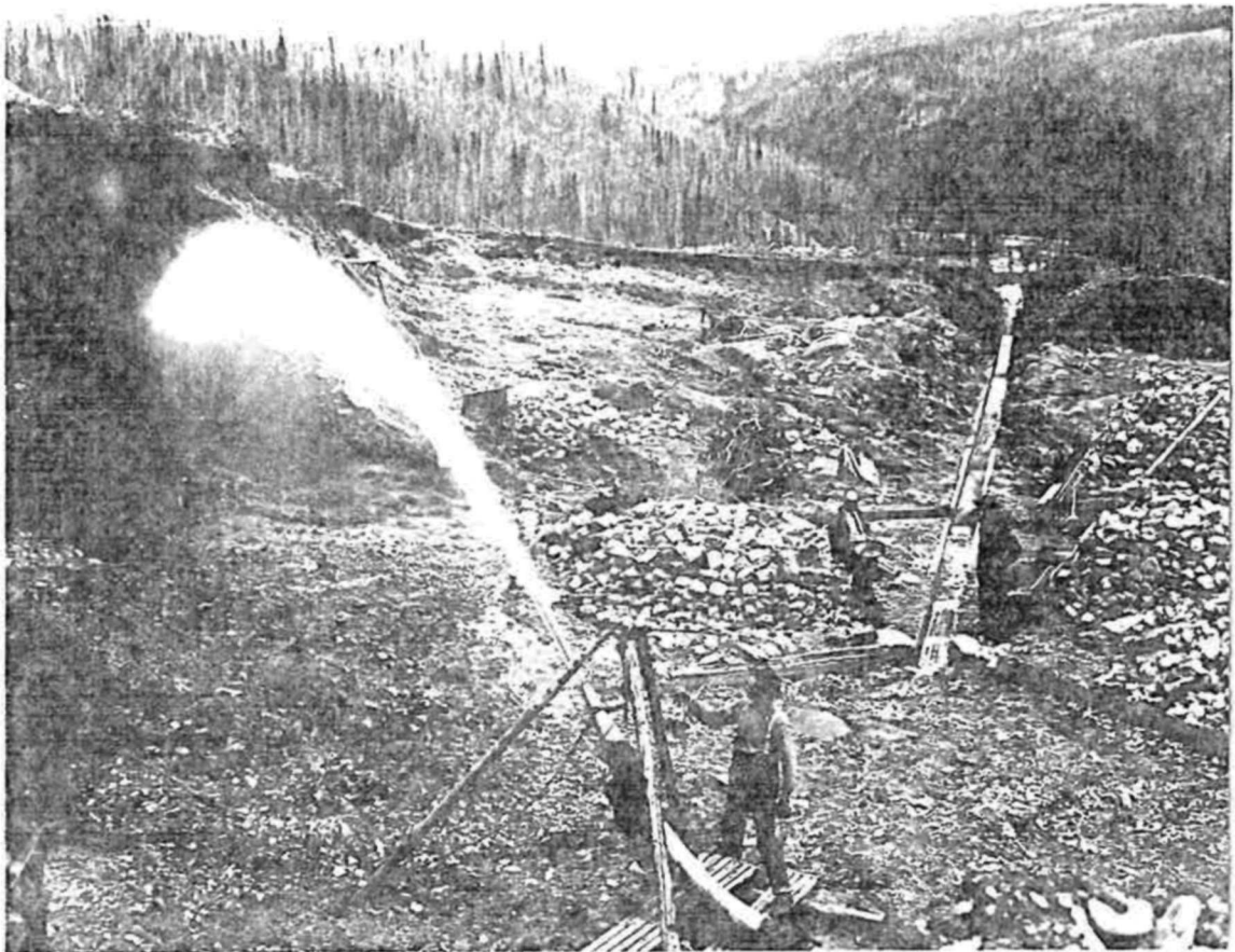
20 Early days of semi-mechanized gold mining in the Klondike: hydraulic thawing of frozen material on a small scale at Flat Creek, ca. 1903. (NA/AN, PA-51480.)
