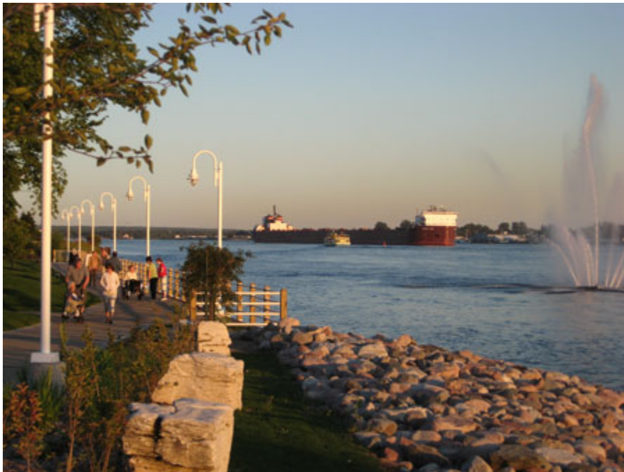
New waterfront walkway, (part of the Hub Trail) Clergue Park area (photo courtesy City of SSM)
