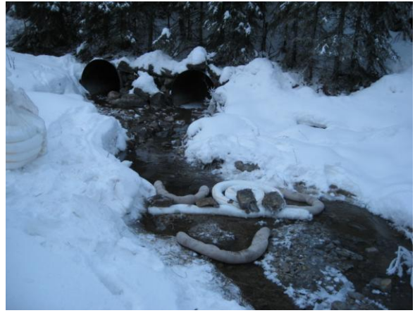
Spill containment on creek by the Field backroad caused by a motor vehicle accident Photo: Parks Canada, K.Schroeder
