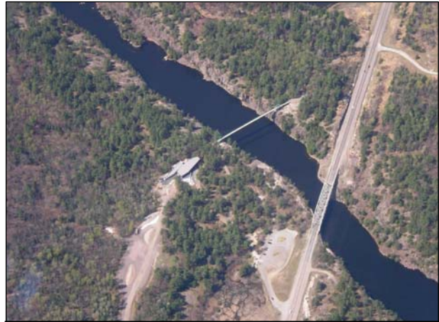
Aerial view of the French River and Visitor Centre at the Highway 69 river crossing. The recreation bridge, highway bridge, the new parking area and the new year-round rest stop are also visible. (Photo courtesy of MNR Staff).
