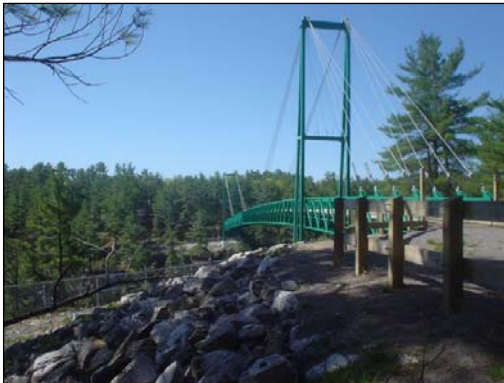
The French River Recreation Bridge spans the French River Gorge, providing a spectacular scenic view of the river and a safe connection between northern and southern Ontario snowmobile trails. (Photo courtesy of MNR Staff).
