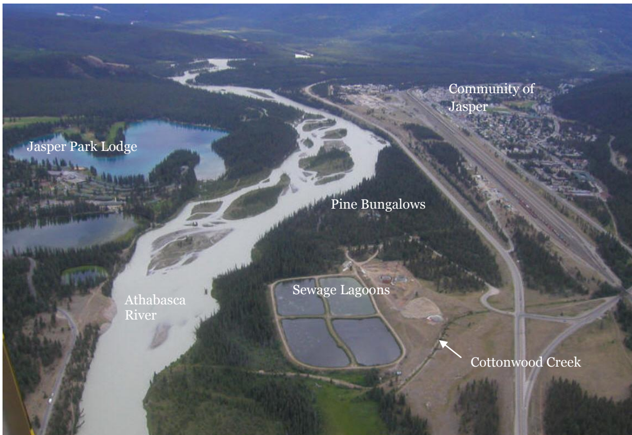
Community of Jasper and wastewater treatment plant before 2003 upgrade
