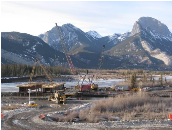
TMX pipeline crossing the Athabasca River Photo: D. Bourdin
