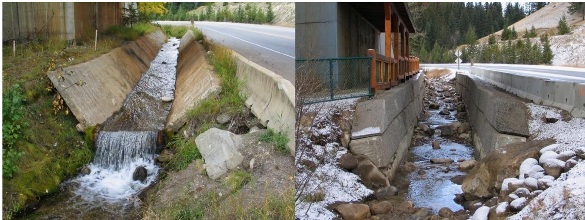
Concrete sluice under railway overpass east of Jasper townsite removed
